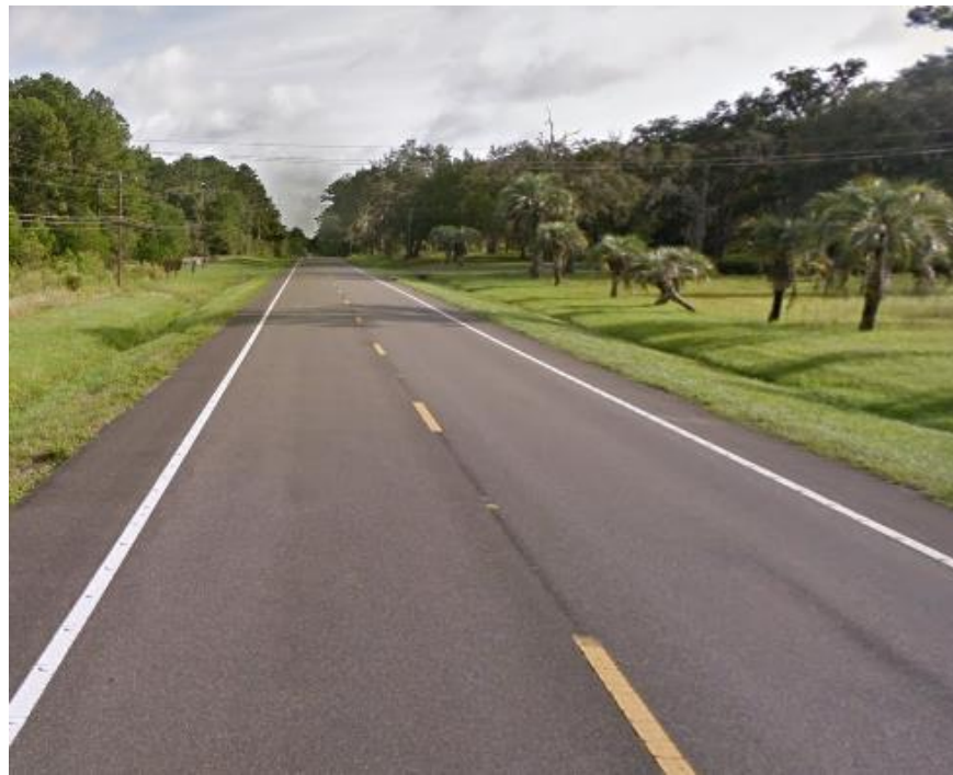
Figure 6-7. 26130000 RCL RPM measurement verification site.
