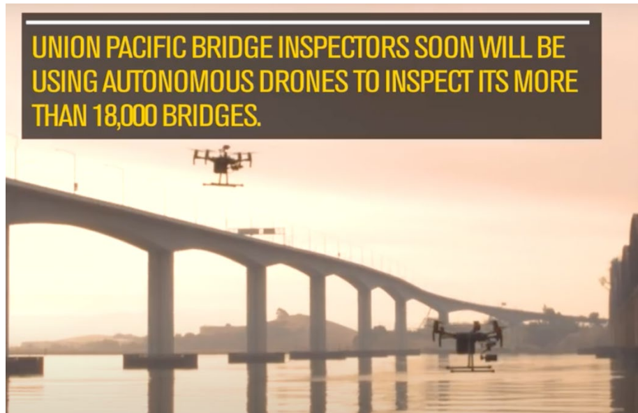
Figure 4.18: UAVs used by Union Pacific to conduct railroad bridge inspections
