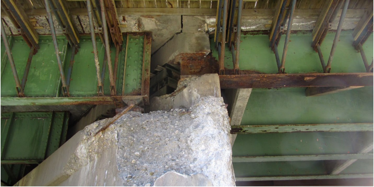
Figure 4.19: Typical condition of aged bridges
