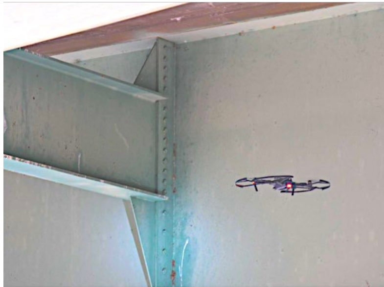
Figure 4.7: DJI Mavic inspecting the Fall River Bridge in Idaho
