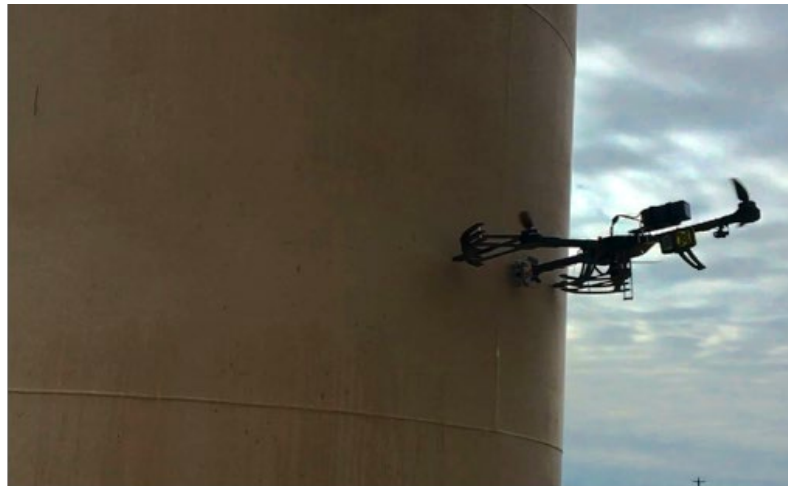
Figure 4.23: Amerapex drone measuring wall thickness
