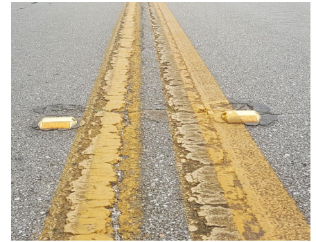
Florida's roadways are lined with millions of raised pavement markers that help drivers follow traffic lanes, especially at night.
