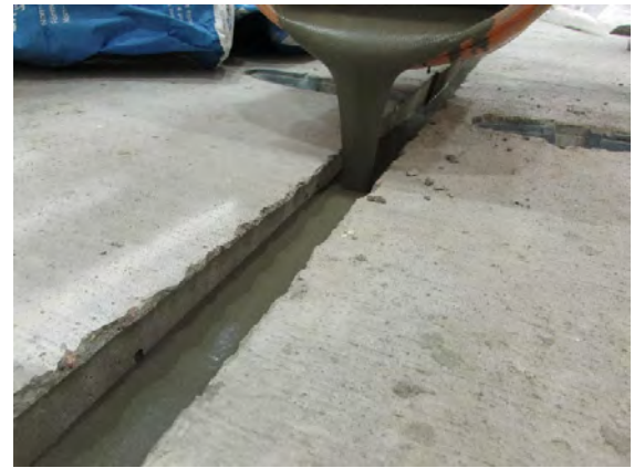
b. Grouting Girder-to-Girder Keyway
