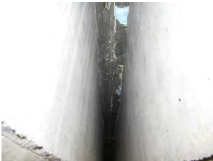
a. Before Testing – Beneath Bridge
