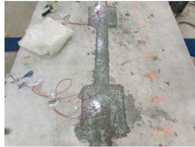
f. Finished UHPC
