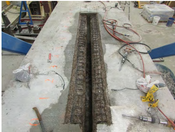
a. Continuous Joint Surface Preparation – Segment I
