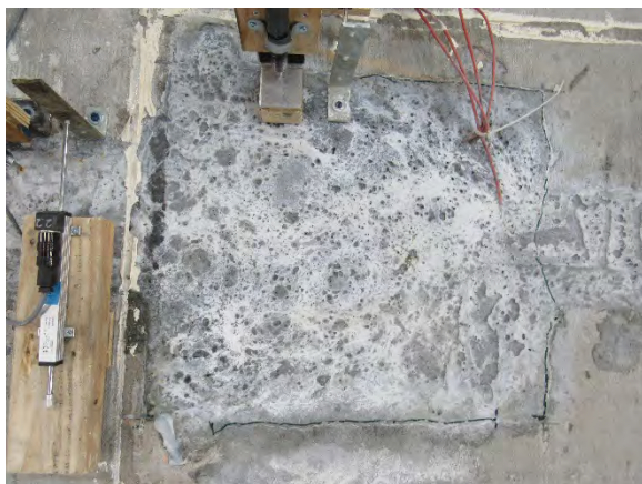
e. UHPC Pocket Joint after Testing
