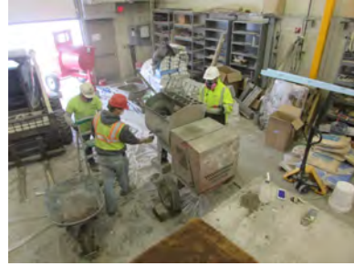
d. Mixing UHPC
