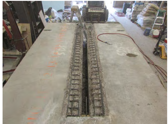
b. Continuous Joint Preparation – Segment II
