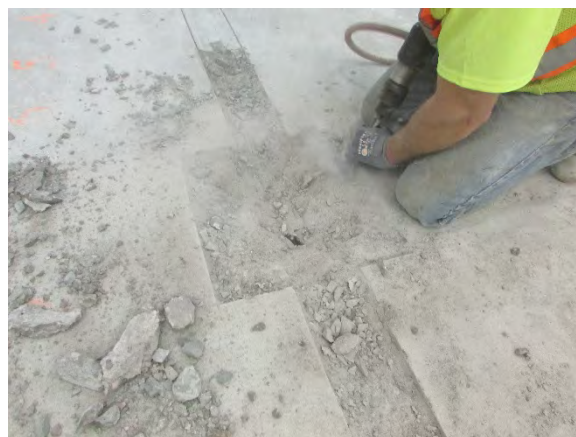
e. Pocket Demolishing
