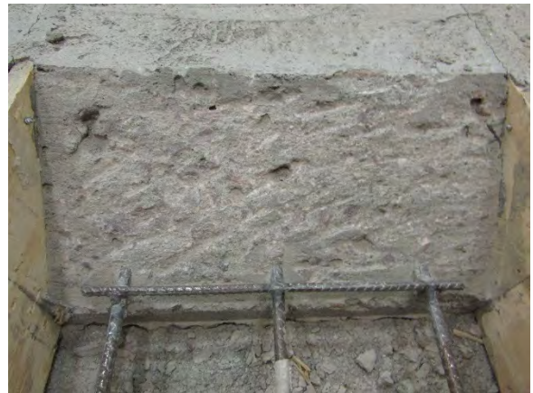
d. Roughened Joint Surface
