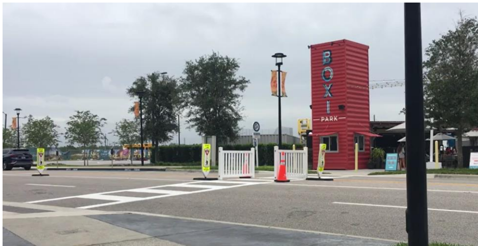
Figure 6-4. EB left-turn bay blocked using fences
