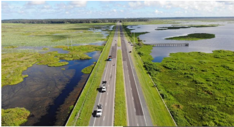
Figure 6-125. Front view showing upstream vehicles changing lanes before approaching the work platoon section
