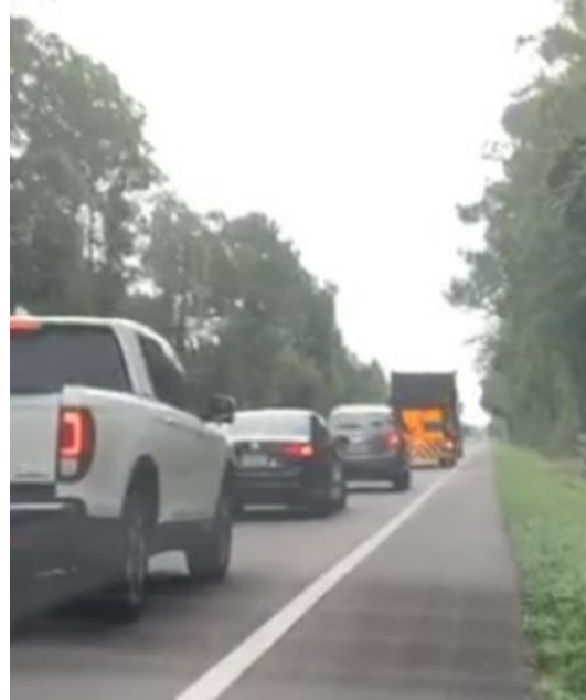
Figure 6-131. Traffic backed up due to slow moving operation on two-lane roadway
