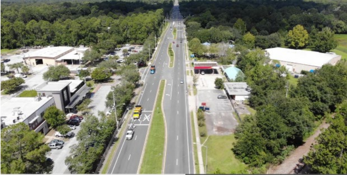
Figure 6-114. Location of Test Site 3 on SR-222 in the Gainesville area
