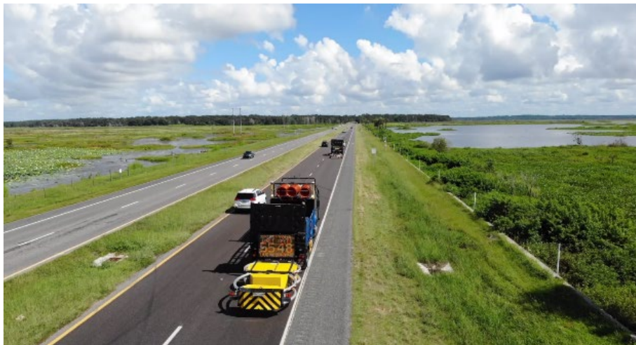
Figure 6-126. View from the back of the work platoon
