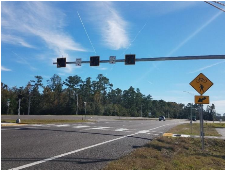
Figure B- 3. Pedestrian hybrid beacon mounted on a mast arm at intersection of Palatka to St. Augustine State Trail and SR 207. Photo courtesy FDOT.
