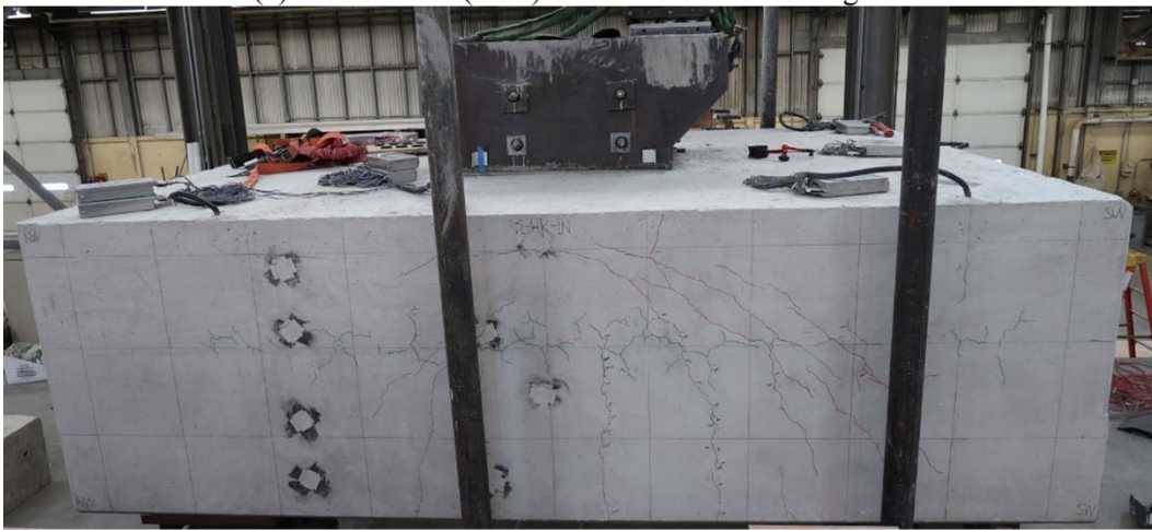
(a) Side surface (west) of VI-HKI after testing
