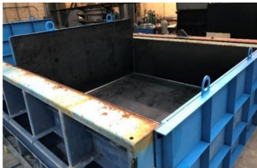
(a) Bottom soffit and side forms
