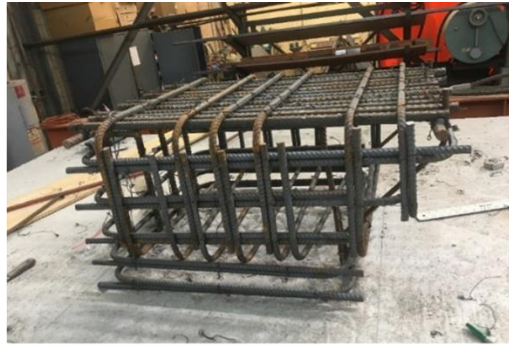
(b) Completed rebar cage
