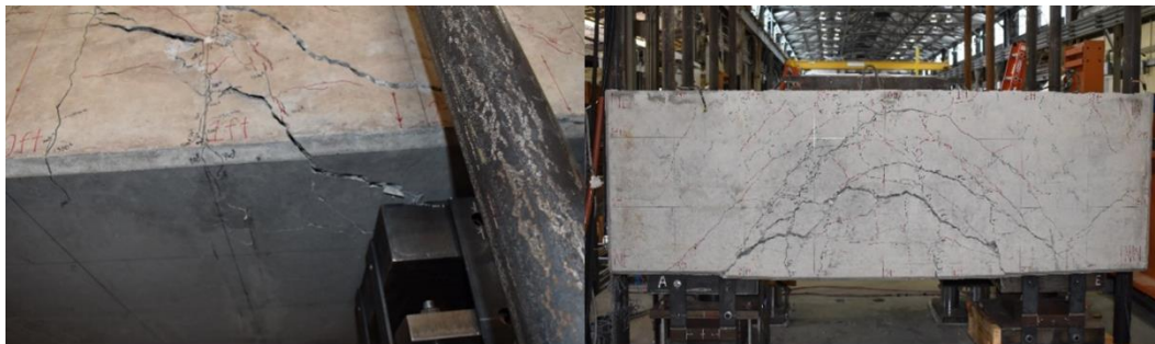
(a) Damage near supports: I-2
