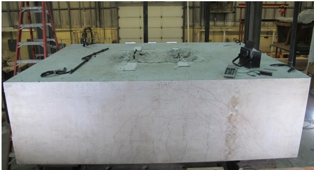
(a) Damage on side surface of footing (west)
