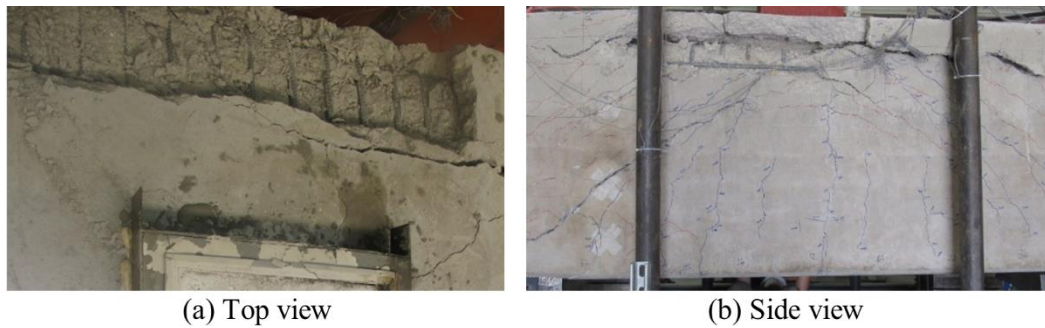
Figure 4.42 Post-failure conditions on top surface of III-9
