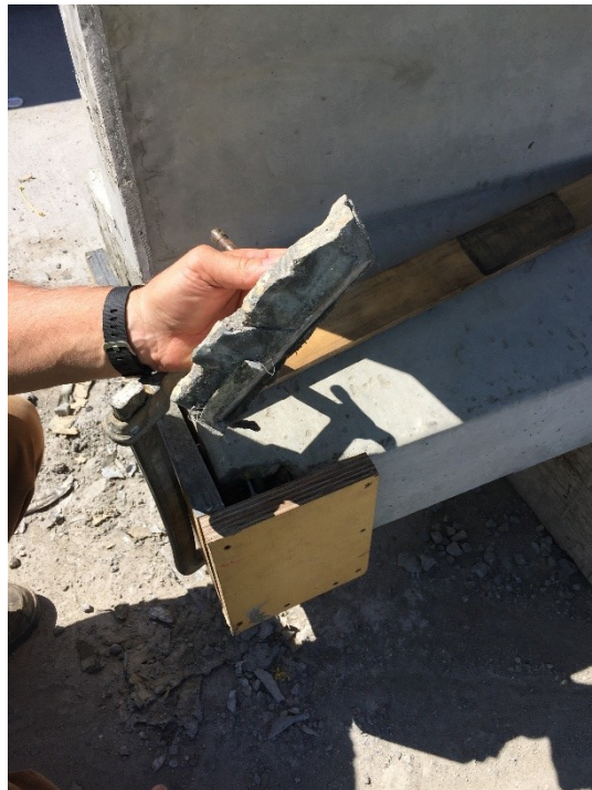
Figure B-3: Image of spalling that occurred during the release of the exterior strands on a 36M girder
