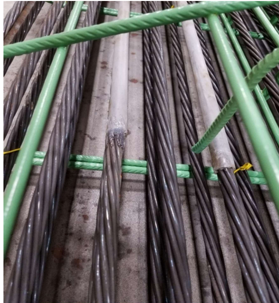
Figure F-9: Silicone sealant applied within the beam form (Photo courtesy of IDOT)
