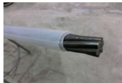
Figure F-8: Double flexible split-sheathing tube method
