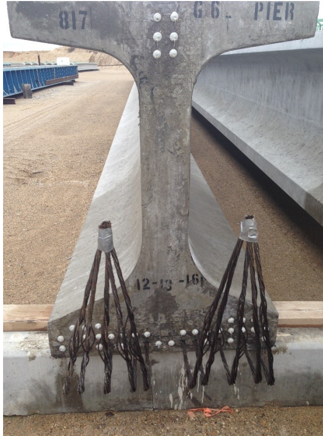
Figure F-1: Exposed strand ends treated with silicone sealant (Photo courtesy of IDOT)
