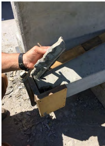
Figure 3-2: Image of spalling that occurred during the release of the outer strands on a 36M girder at County Materials in Roberts, WI
