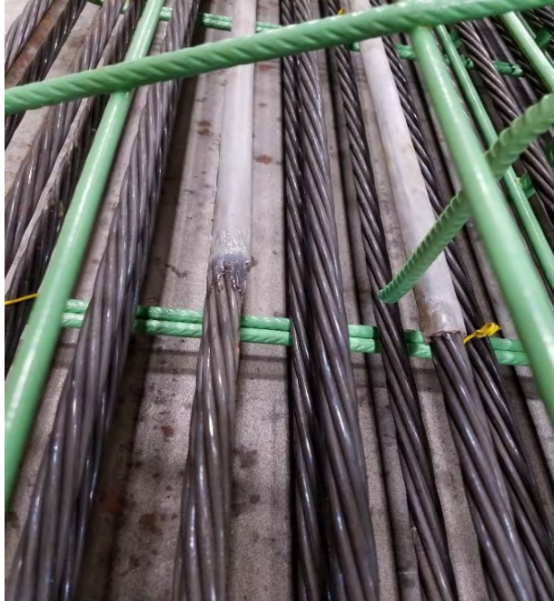
Figure 5-5: Silicone sealant applied within the beam form (Photo courtesy of IDOT)
