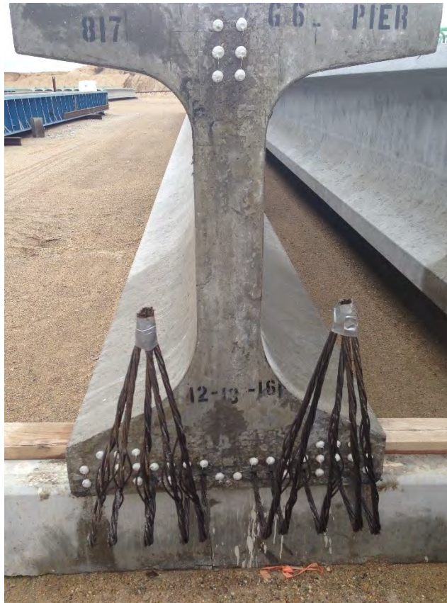
Figure 5-1: Exposed strand ends treated with silicone sealant (Photo courtesy of IDOT)
