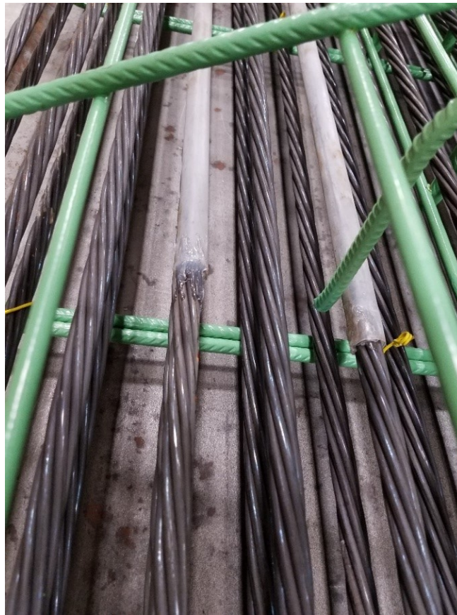
Figure F-4: Silicone sealant applied within the beam form (Photo courtesy of IDOT)
