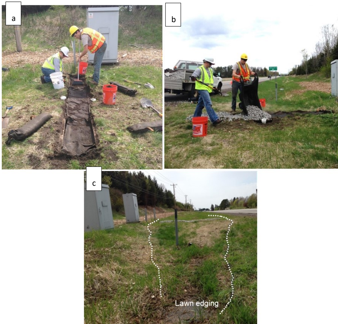
Figure 4.1. Maintenance performed at the ditch check site in May 2017. The topsoil and sod covering the filter insert section were removed (a & b), and lawn edging (highlighted by white dashed line) was installed along the ditch check (c).
