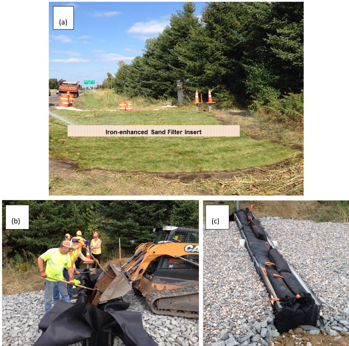
Figure 2.3. (a) Photograph of the iron-enhanced ditch check (Ditch Check 2) along CR 15 (formerly TH 5) in Stillwater, Washington County (Photograph by P. Natarajan, 2014). Approximate location of the filter insert in the ditch check is shown. (b) Photograph taken during construction in 2014 shows the placement of filter media into a single geotextile fabric that was wrapped to form the filter insert core inside the filter cage, and (c) Photograph shows the completed filter insert.
