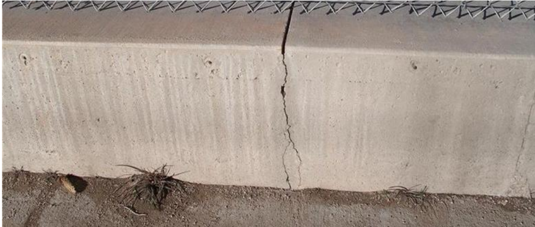
Figure 5. Crack vs concrete groove ( https://www.concretenetwork.com ).
