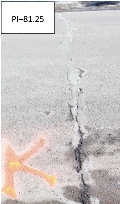
(b) Site K: 2nd St.: 24-26 AE, Duluth; Crack Sealing Year – 2016
