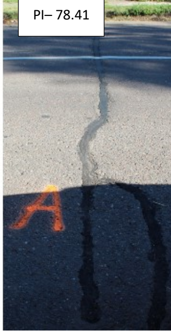
(e) Site A: 3rd St:21st AE to 1st AE, Duluth; Crack Sealing Year - 2014
