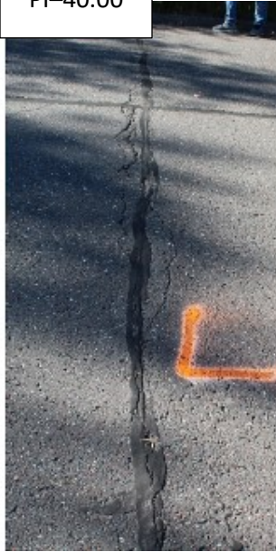
(a) Site L: 1 st St.: 24- 26 AE., Duluth; Crack Sealing Year – 2016; **Snow Cover
