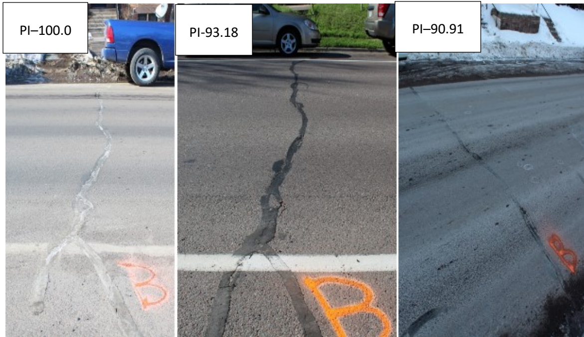
Duluth; Crack Sealing Year – 2014
