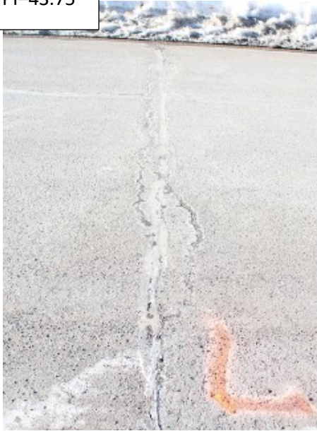
(a) Site L: 1 st St.: 24- 26 AE., Duluth; Crack Sealing Year – 2016; **Snow Cover
