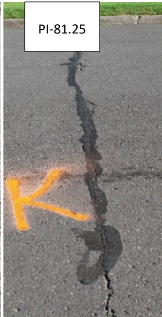
(b) Site K: 2nd St.: 24-26 AE, Duluth; Crack Sealing Year – 2016
