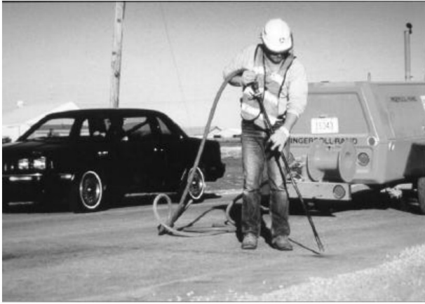
Figure 2.4: Airblaster Being used to Clean a Crack (after, Smith and Romine, 1999)
