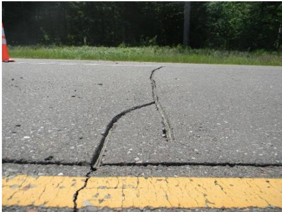
Figure 2.16: Routed Crack After Cleaning
