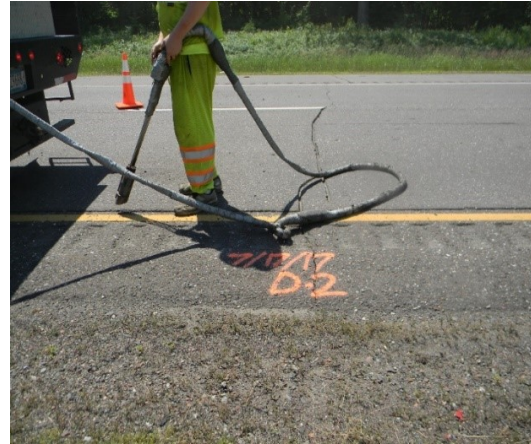
Figure 2.5: Air lance being used to Clean a Crack
