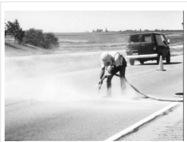
Figure 2.6: Sandblaster Being Used to Clean a Crack (after, Smith and Romine, 1999)
