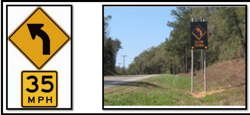
Figure 1.1 Examples of horizontal curve warning signs: on the left a static sign, on the right a dynamic curve speed warning sign.
