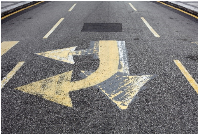
Figure 3-2. Example of overlapping pavement markings
