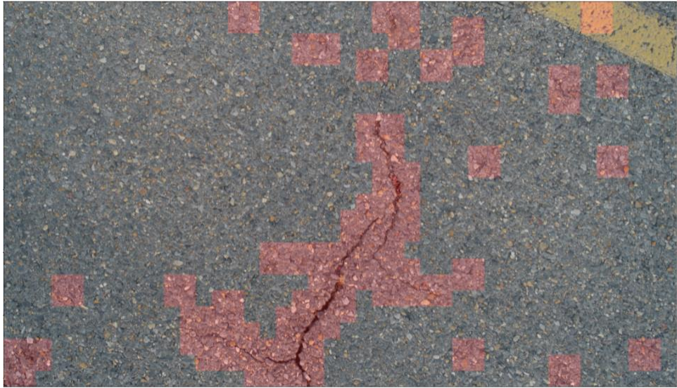
Figure 19. Detection of asphalt pavement crack without identifying boundary markers as false cracks
