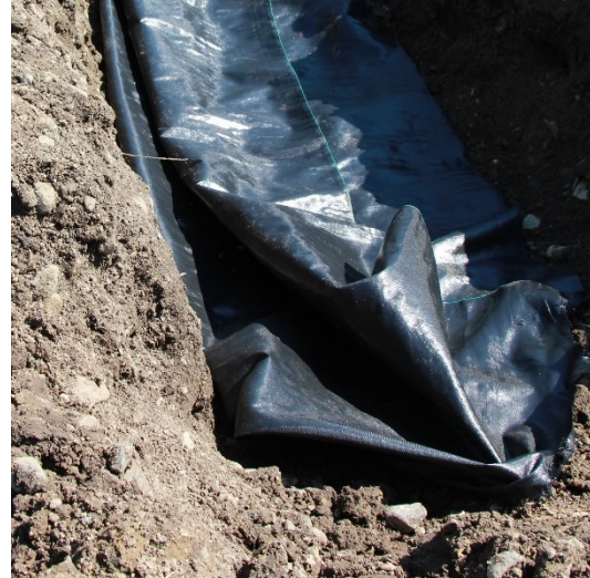
Figure 6.4. Permeable membrane sleeve and geomembrane placed at site to protect underdrain from clogging.
