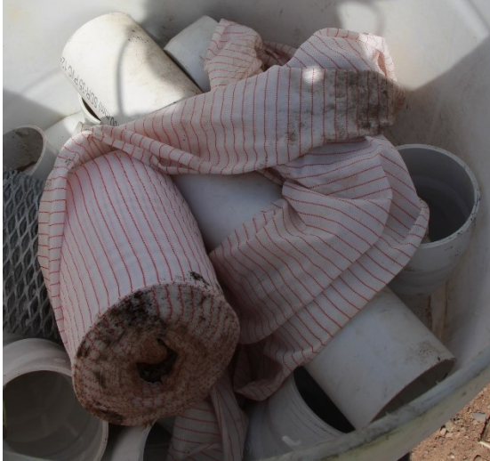
Figure 6.4. Permeable membrane sleeve and geomembrane placed at site to protect underdrain from clogging.
