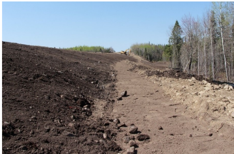
Figure 6.3. Bioswale construction at midpoint of hillside.
