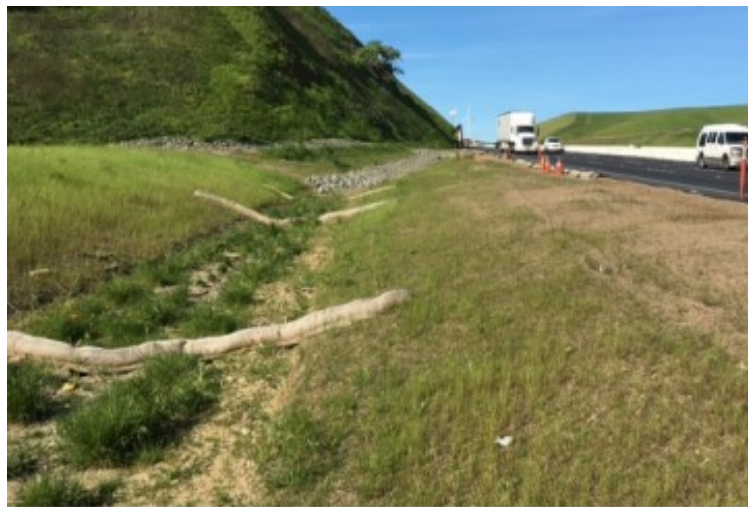
Figure 2.16. Vegetated swale with temporary check dam (Caltrans, 2017).
