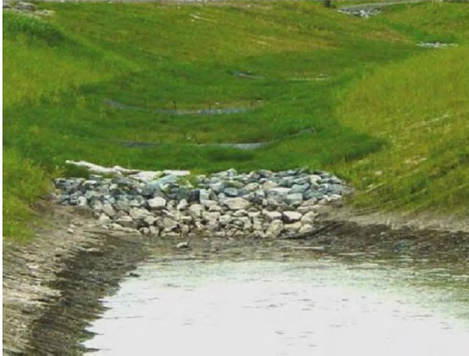
Figure 2.14. Bioswale with designed outflow into a detention pond (adapted from ODOT, 2014).
