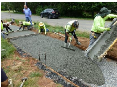
Placement and finishing operations
