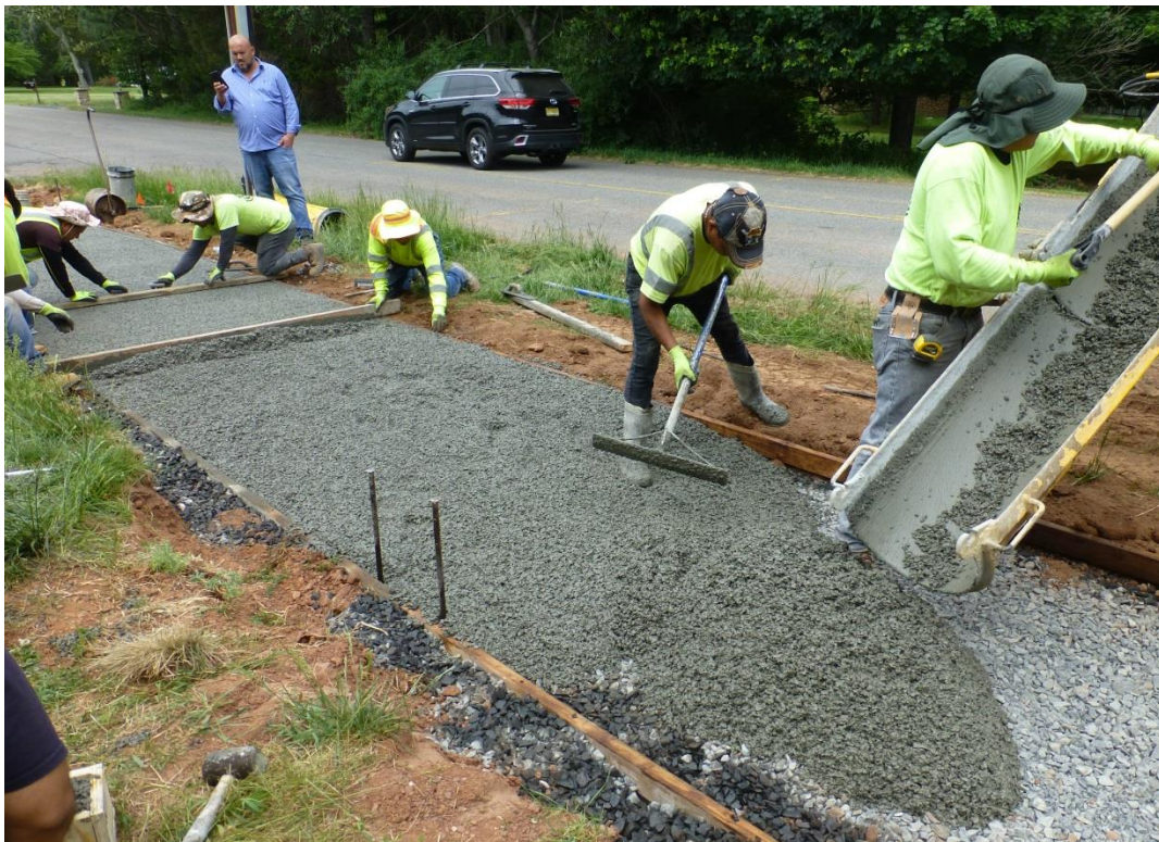
Figure 17. Porous concrete placement
