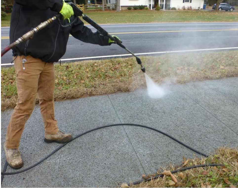
Figure 29. Pressure washing with water pressure ranging from 3000 psi to 3500 psi
