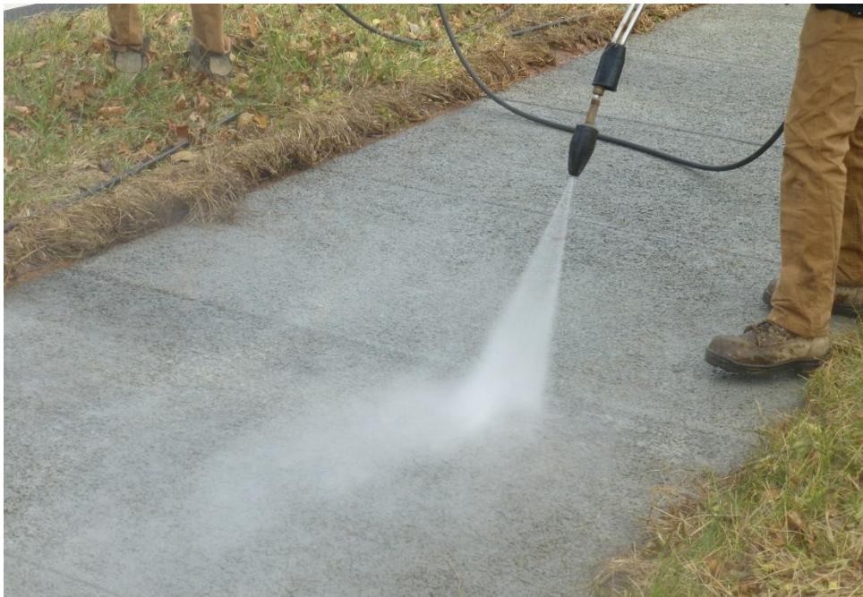
Figure 30. Pressure washing with water pressure ranging from 3000 psi to 3500 psi
