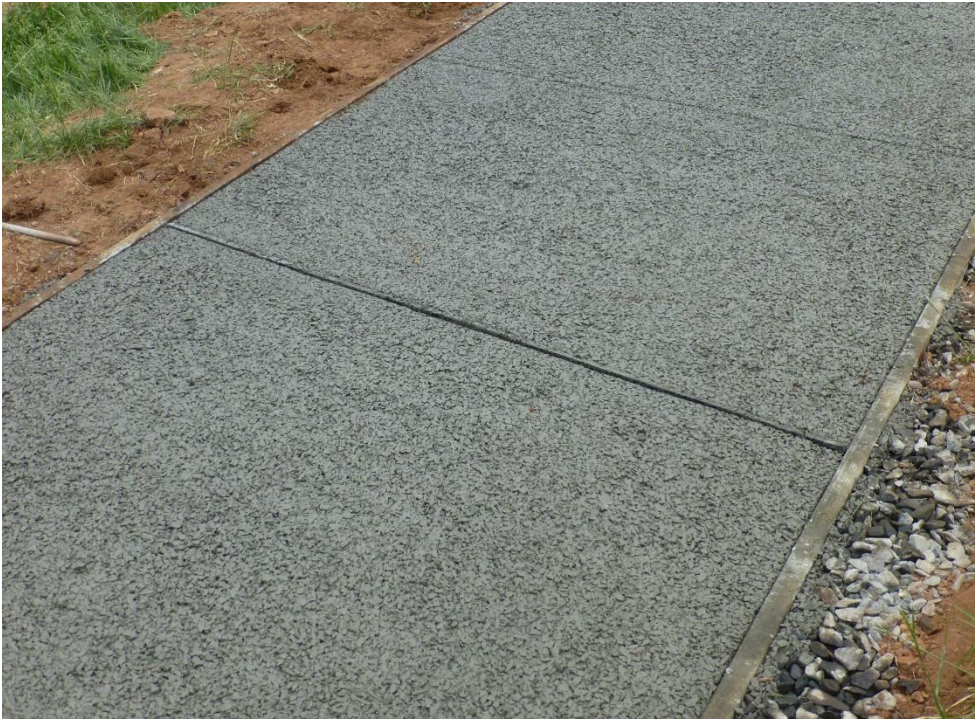
Figure 18. Finished porous concrete surface
