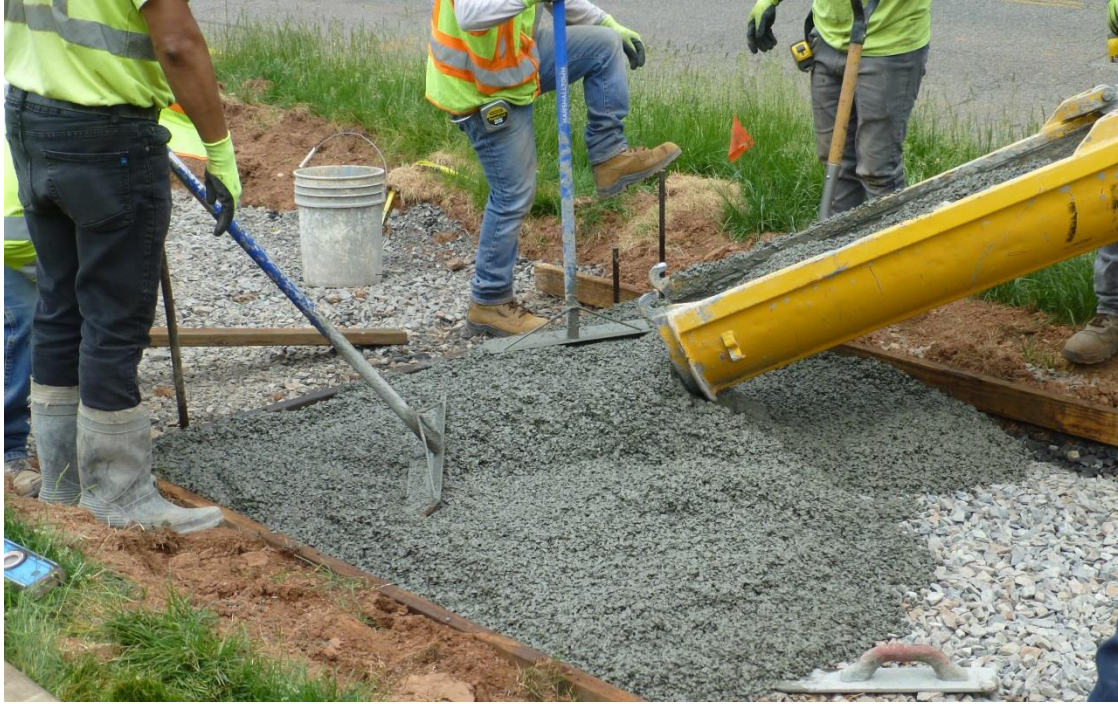
Figure 16. Discharging porous concrete from ready mix truck
