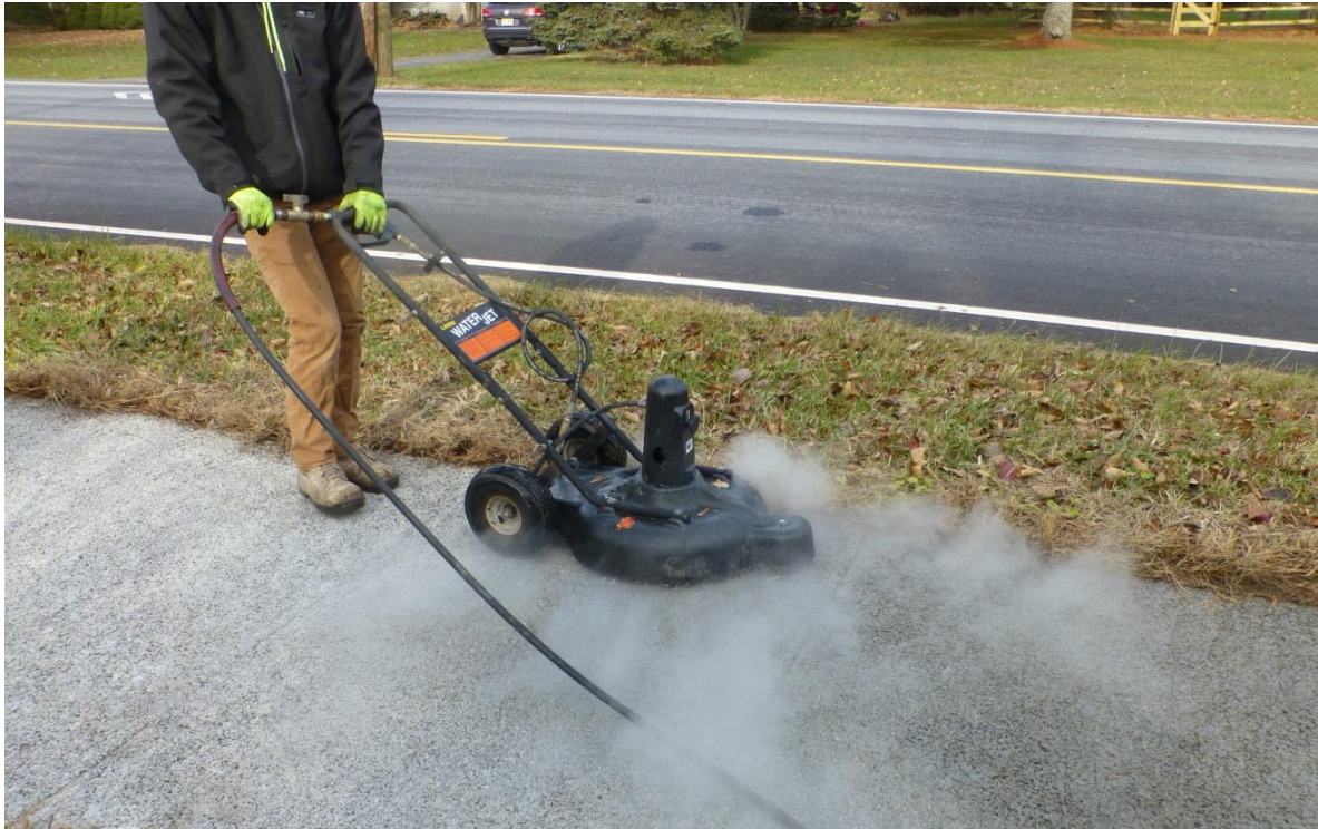
Figure 28. Pressure washing with water pressure of about 2000 psi
