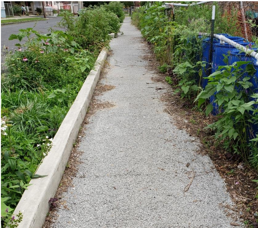
Figure 4. Porous concrete surface of well-maintained porous concrete sidewalk (Location B)
