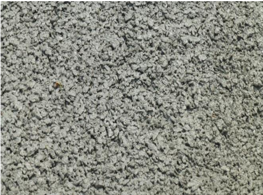
Figure 19. Closeup of finished porous concrete surface
