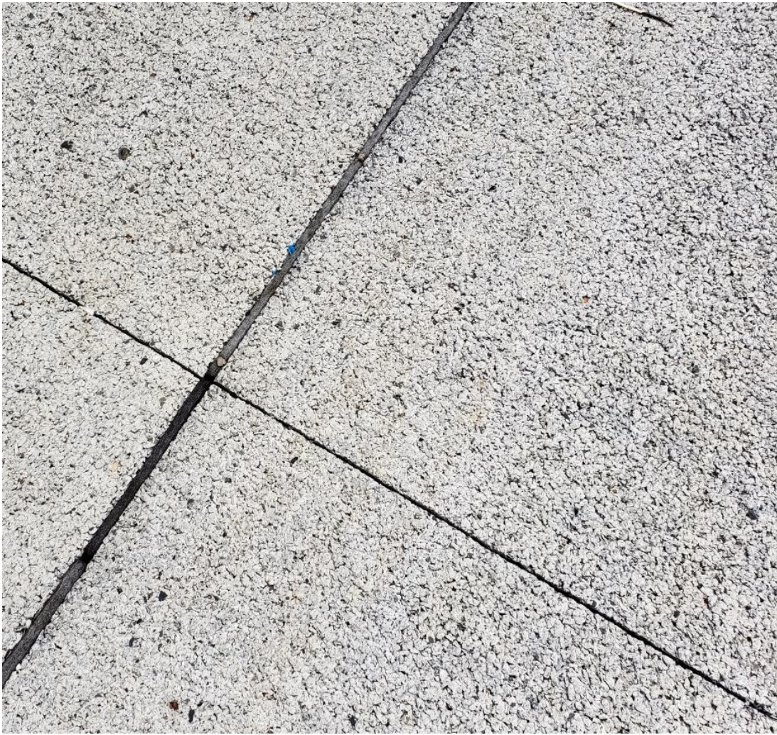
Figure 3. Porous concrete surface of well-maintained porous concrete sidewalk (Location A)
