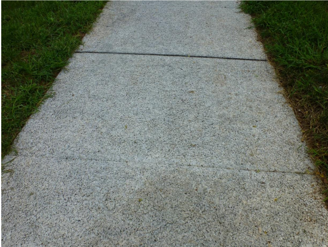
Figure 21. Baseline photo of finished sidewalk surface
