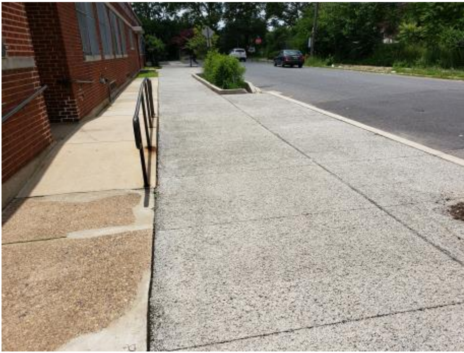
Figure 2. Porous concrete surface of well-maintained porous concrete sidewalk (Location A)
