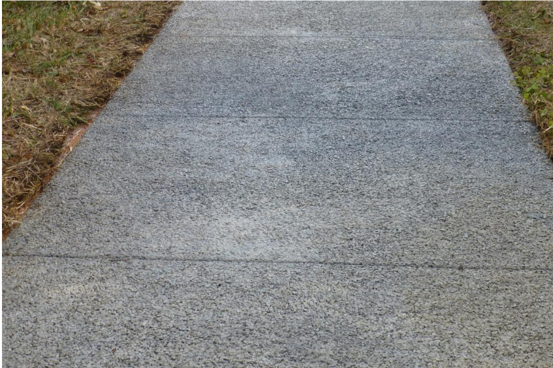
Figure 31. Finished porous concrete sidewalk after pressure washing
