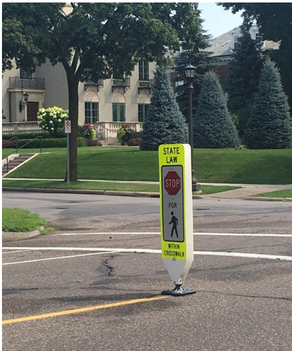
Figure 3.12 Single in-street sign (R1-6) on yellow centerline at Summit and Chatsworth
