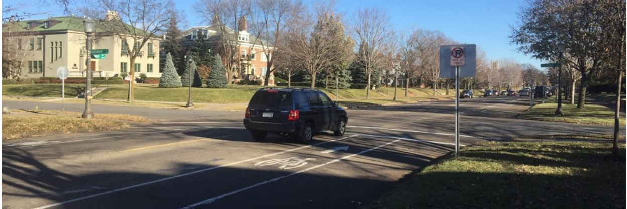
Figure 4.5 The crosswalk at Summit & Chatsworth, a two-lane with bike lane and parking lane on both sides of the roadway.
