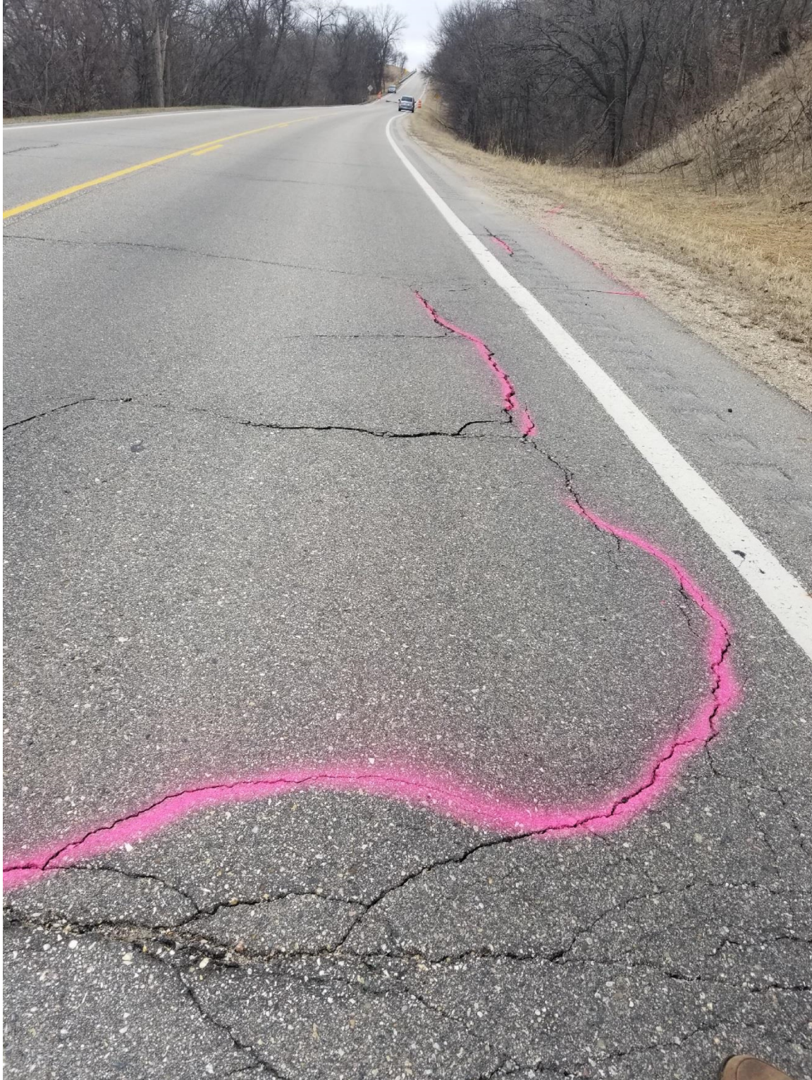
Figure 18. Cracks occur as far as 1000 feet from one another along TH67. Photo: Nick Bradley, WSB.
