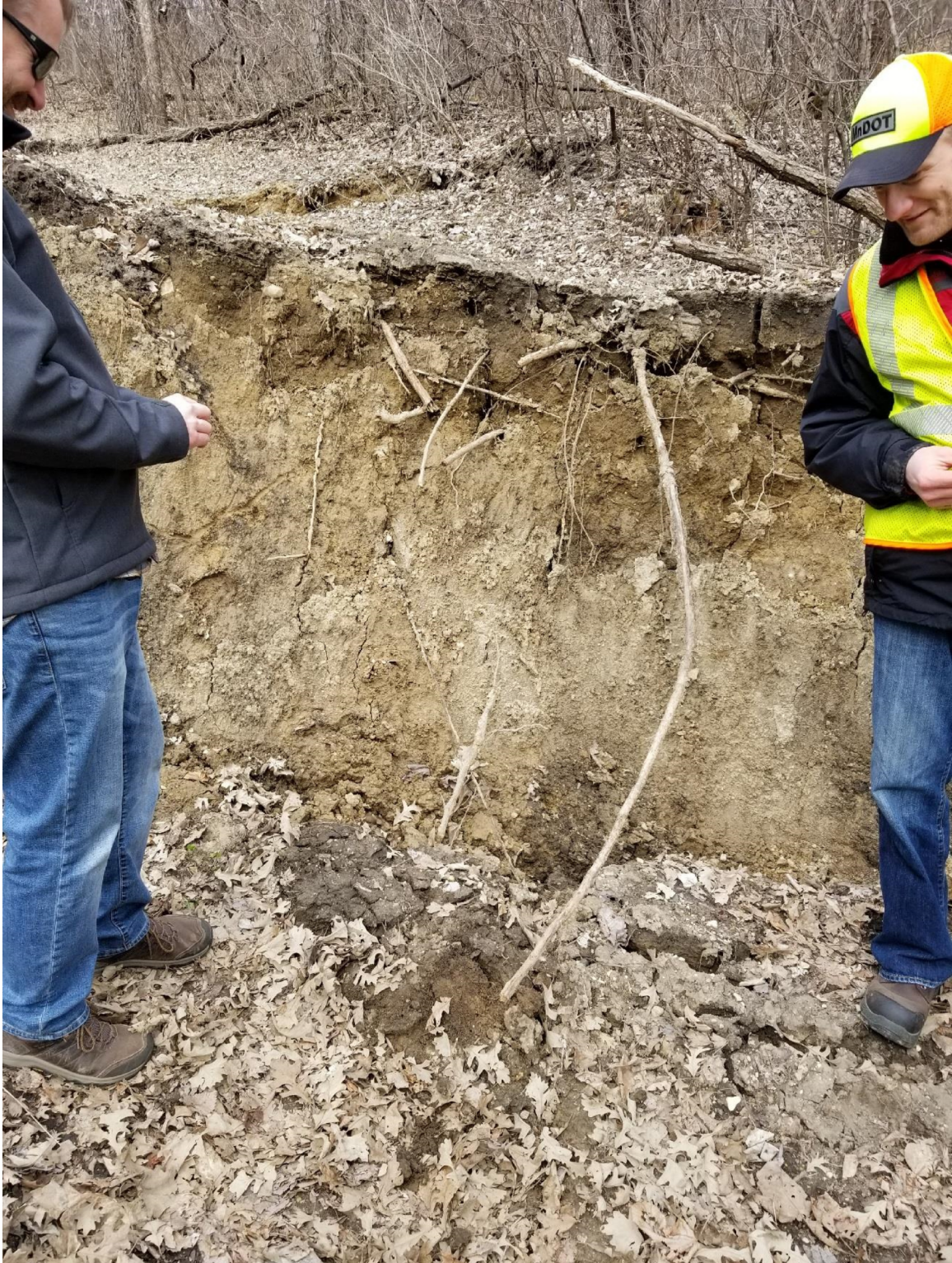
Figure 20. Scarp in floodplain causes the trail to become unusable. Photo: Nick Bradley, WSB.
