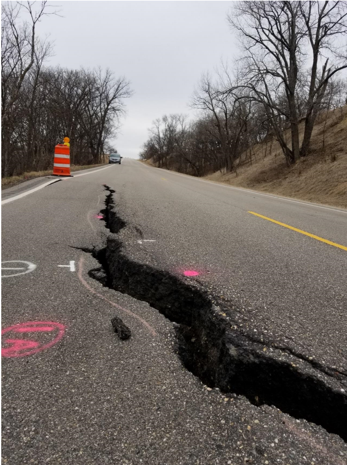
Figure 17. Crack in TH67 causes road closures and indicates deep-seated slope failures. Photo: Nick Bradley, WSB.
