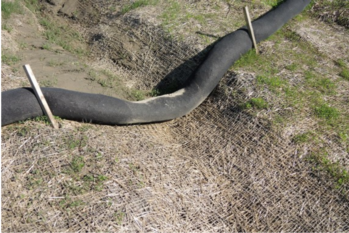
Figure 32 Product chosen could not handle the flow at this location. Another sediment control log that could withstand higher flows would be a more appropriate choice.
