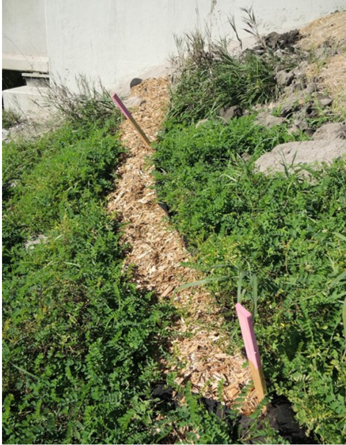
Figure 33 Product required maintenance prior to its current state. Replacement at the time of the photo is required to continue controlling erosion at the site.
