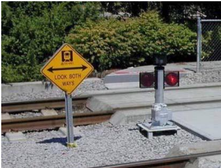
Figure 28. Low-mount flashing light signal, Tri-Met, Portland, OR
