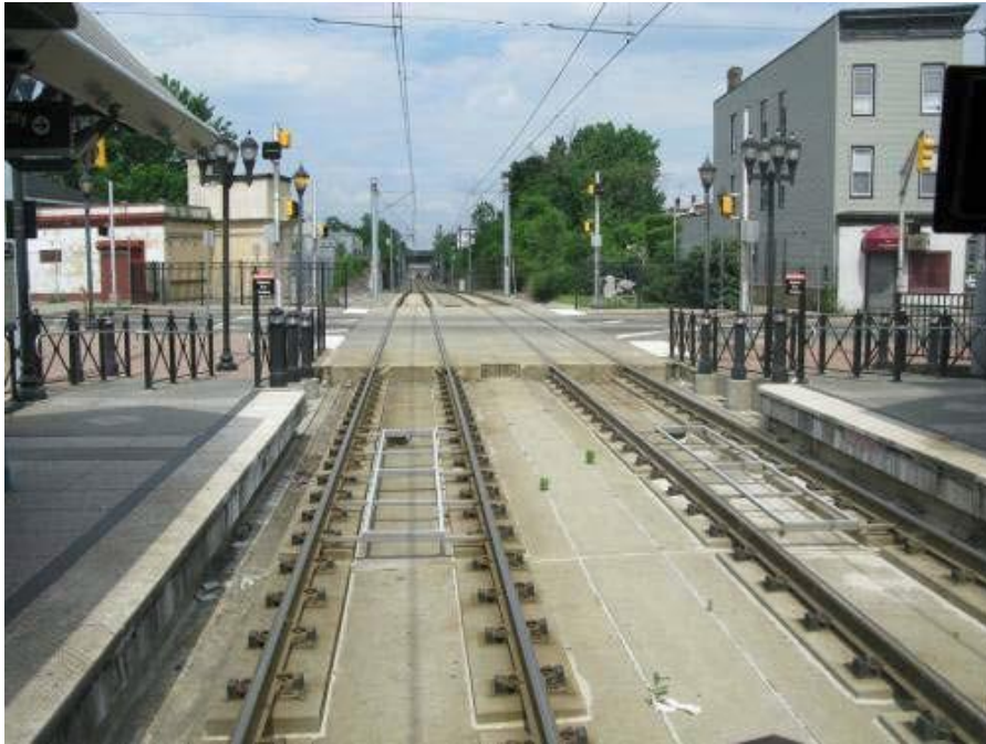
Figure 8. Typical type b.1 alignment New Jersey Transit, NJ
