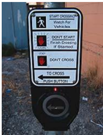
Figure 38. Pedestrian sign integrated with pedestrian pushbutton
