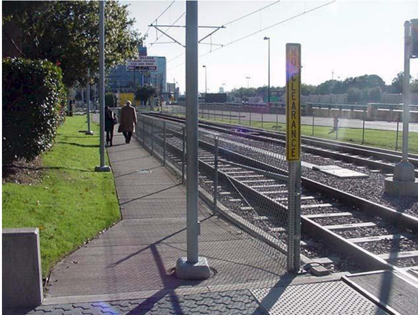
Figure 49. Pedestrian fencing, DART, Dallas, Texas
