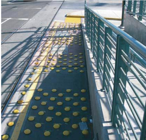
Figure 65. Raised yellow markers to warn pedestrians to stay off of the narrow strip of pavement between LRT tracks and the median station, MUNI, San Francisco, CA
