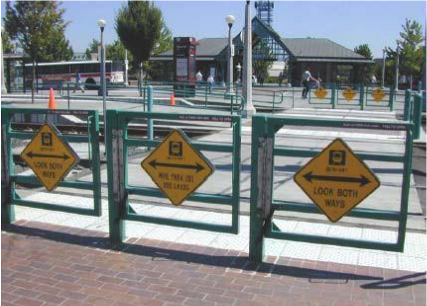
Figure 45. Pedestrian swing gates, Tri-Met LRT, Portland, OR
