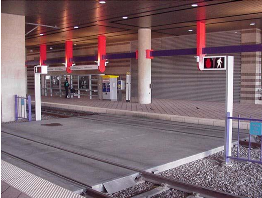
Figure 36. Pedestrian signals, DART, Dallas, TX
