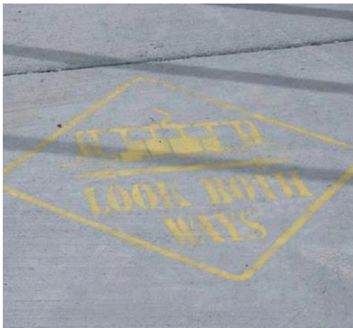
Figure 61. Painted “LOOK BOTH WAYS” on concrete pedestrian path before crossing, UTA, Salt Lake City, UT
