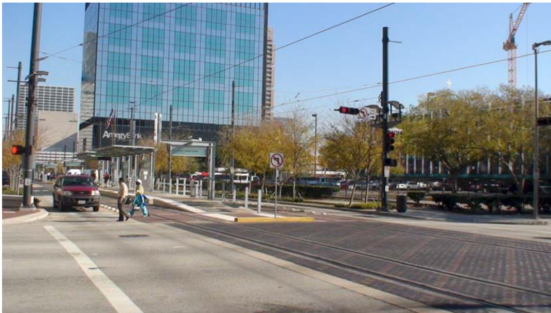
Figure 59. Colored, textured concrete marking of LRV track area, Houston Metro, TX
