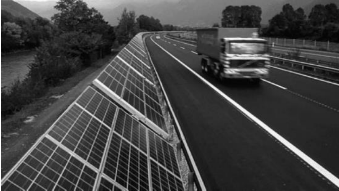
Figure 9. Photovoltaic noise barrier along the A13 highway in Switzerland (20).
