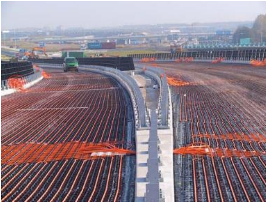
Figure 4. Asphalt solar collector system under construction on a bridge in Rotterdam (14)
