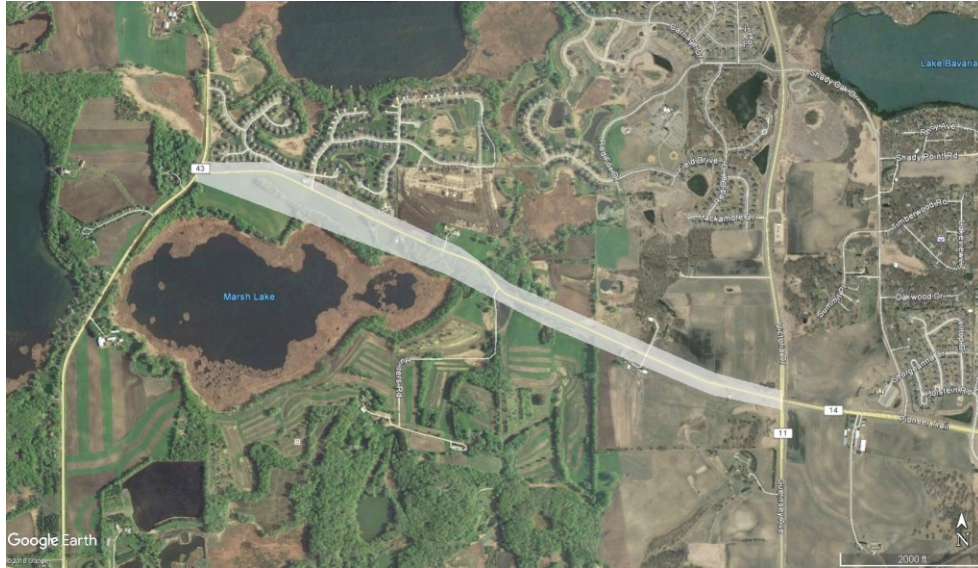
Figure 2-1: Marsh Lake Road UAV Survey Extents.
