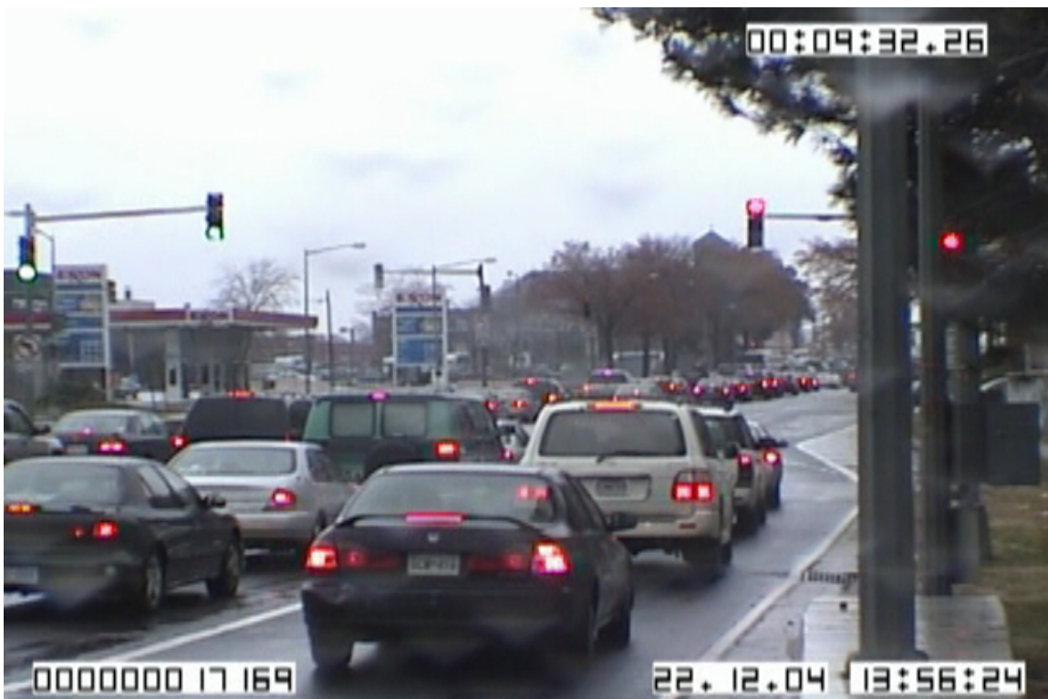
Figure A8-3 – At South Capitol and I (Eye) Street Intersection, the driver can see the signal faces on the left prior to those on the right, which the driver should obey
