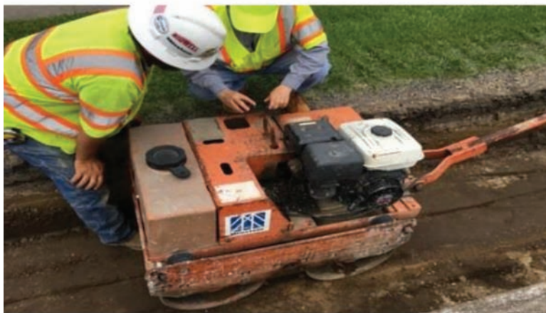
(b) Pavement patching
