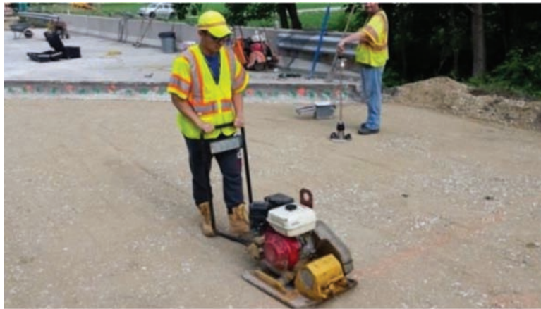
(a) Bridge approach
