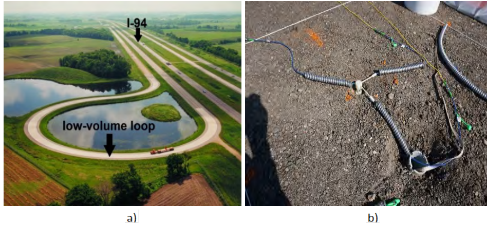
Figure 2.2 (a) MnROAD facility and (b) the sensor installation scene
