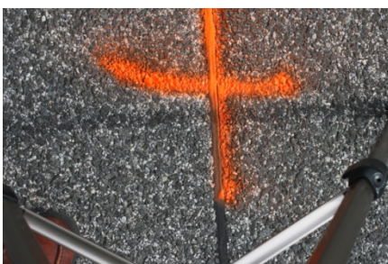
Figure 8.10 (i – vii): Conditions of HMA Overlay Longitudinal Saw-Cuts
