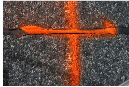
Figure 8.9 (a – o): Conditions of HMA Overlay Transverse Saw-Cuts
