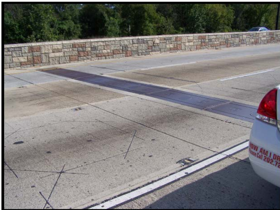
Figure 3: New York Avenue WIM Site
