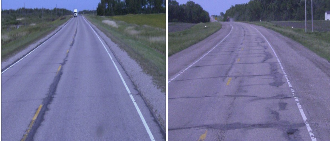
Figure 2.3: Physical meaning of Ride Quality Index (RQI). a) RQI = 3.2 and b) RQI = 1.6
