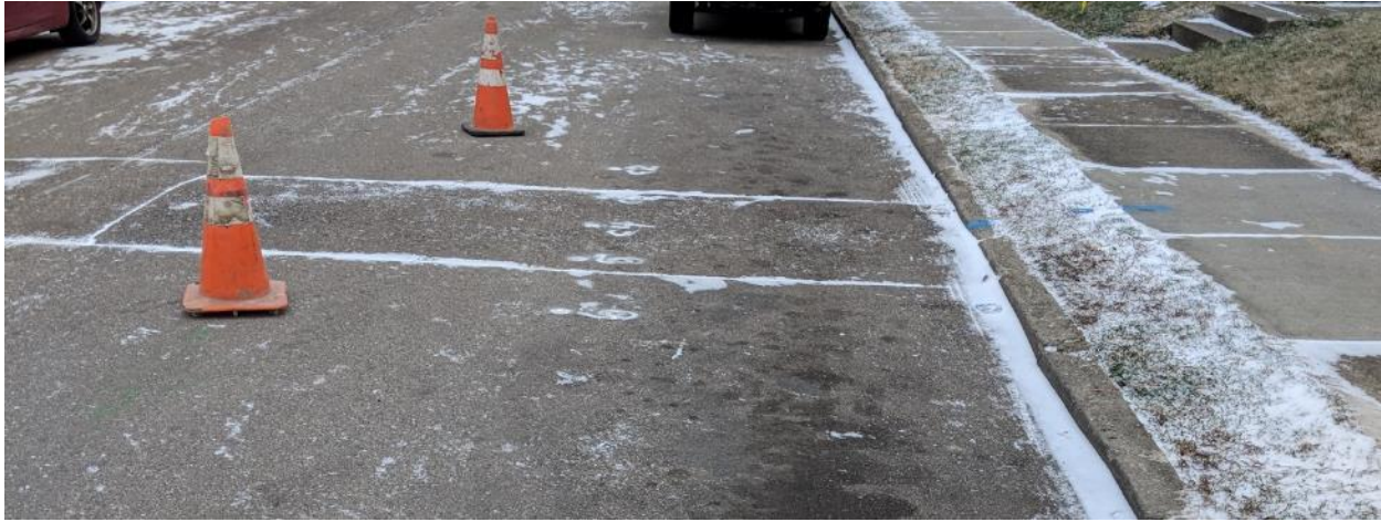
Figure 40 Repair on 66 S. Sperling Ave.
