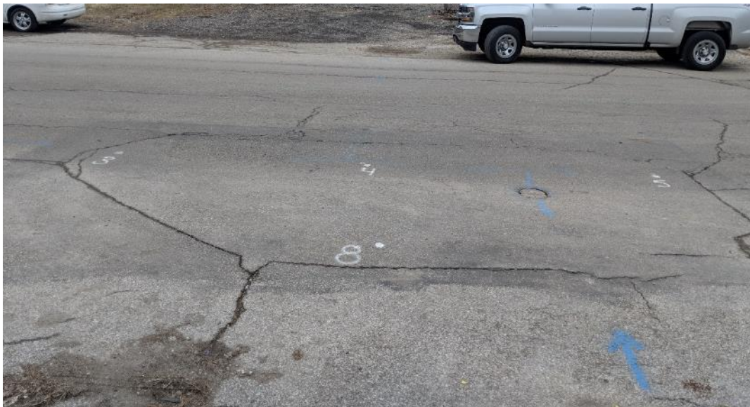
Figure 39 Repair at 1734 Old Leonard Ave.
