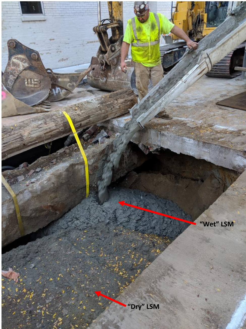
Figure 23 Observed open cut utility repair in progress, City of Cleveland.
