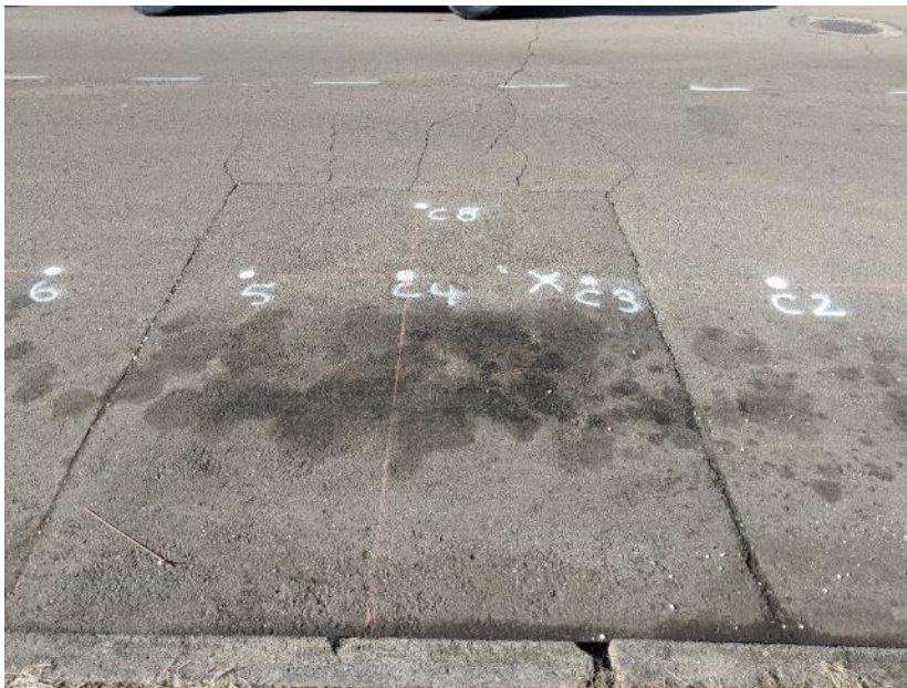
Figure 41 Repair on 74 S. Sperling Ave.
