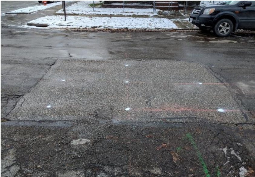
Figure 30 Repair on Woodbridge Ave.
