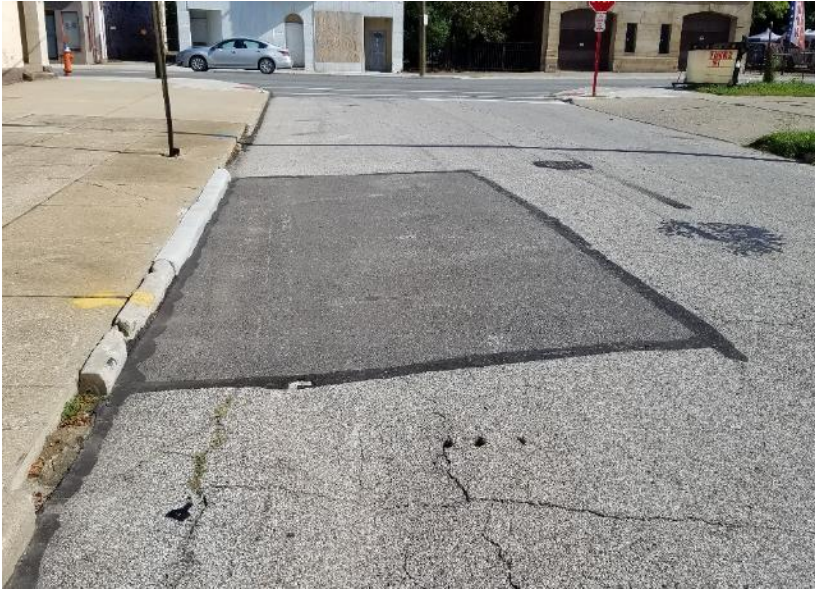
Figure 28 Repair on Pepper Ave.
