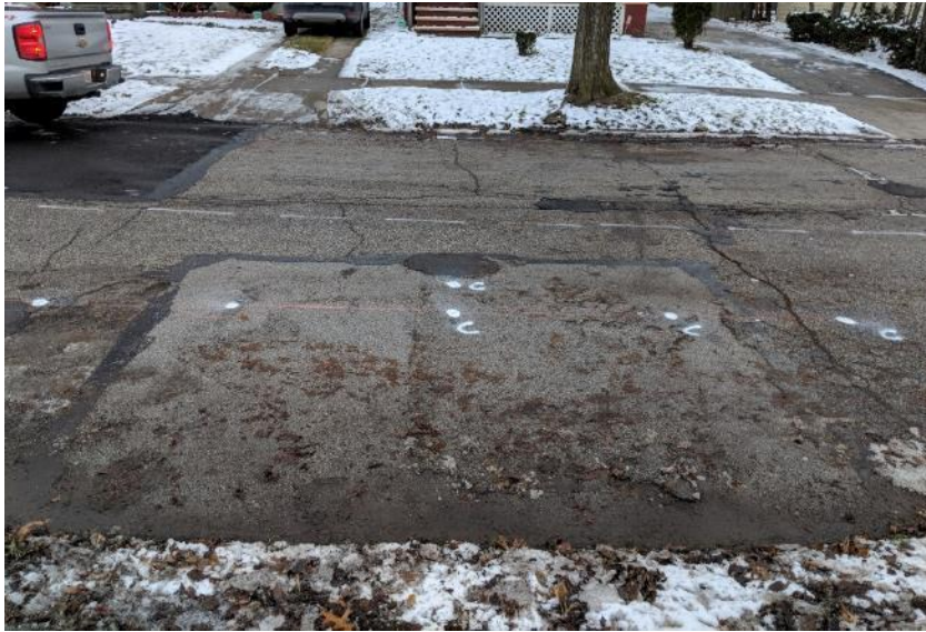
Figure 32 Repair on Terminal Ave.
