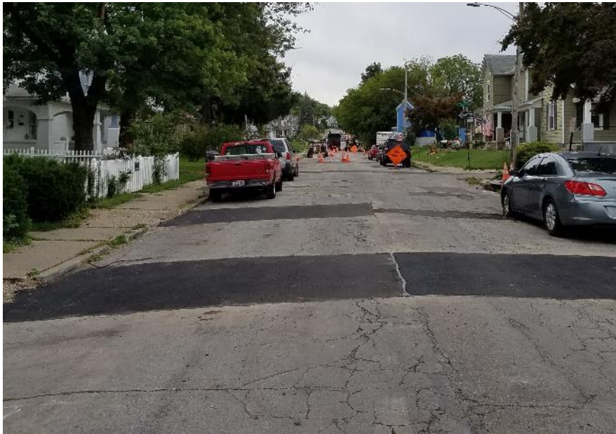
Figure 27 Example of completed permanent repair, City of Dayton.
