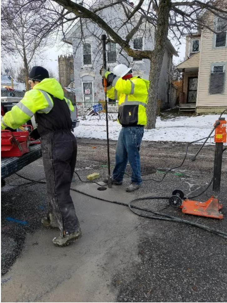
Figure 8 Sampling of base or backfill material.
