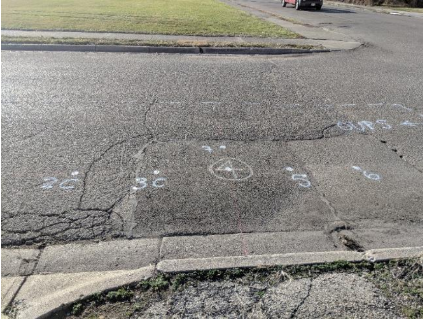
Figure 42 Repair on N. Torrence at Springfield.
