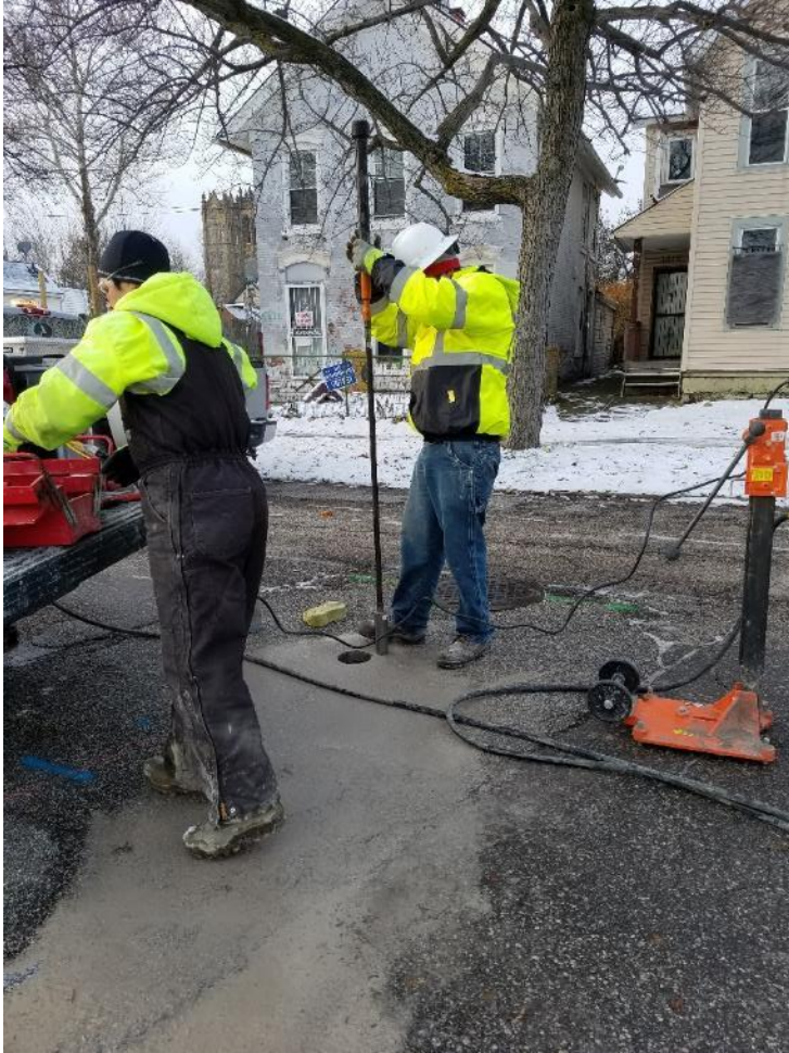
Figure 53 Sampling of base or backfill material.
