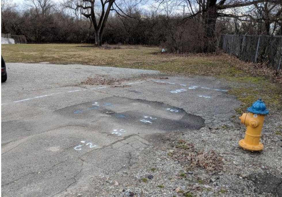
Figure 44 Repair on 316 Urbana Ave.
