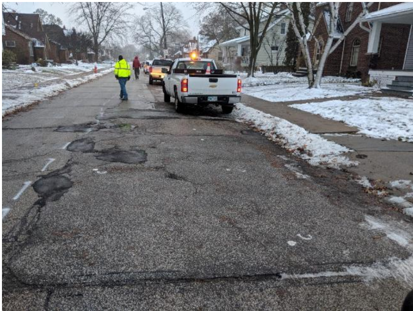
Figure 33 Repair on Valleyview Ave.
