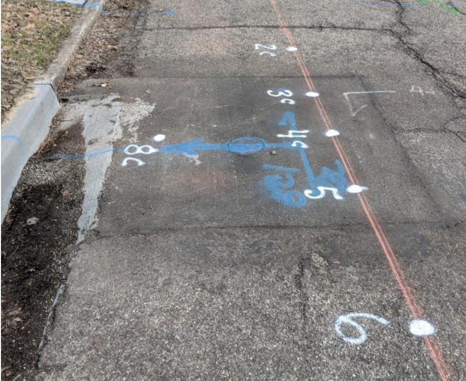
Figure 35 Repair at 50 E. Jeffrey Place.
