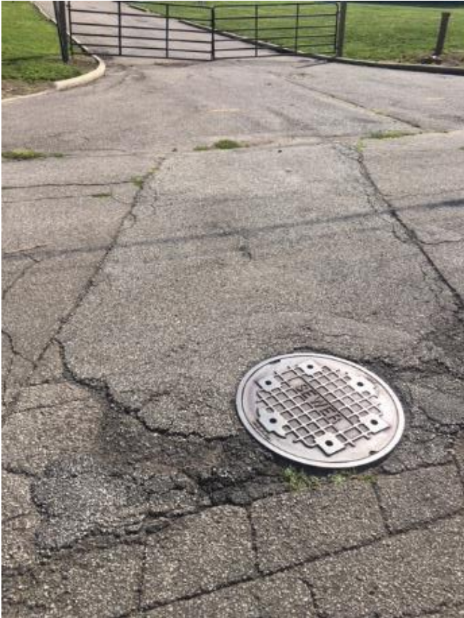
Figure 31 Repair on E. 45 Street Location (Courtesy of City of Cleveland).
