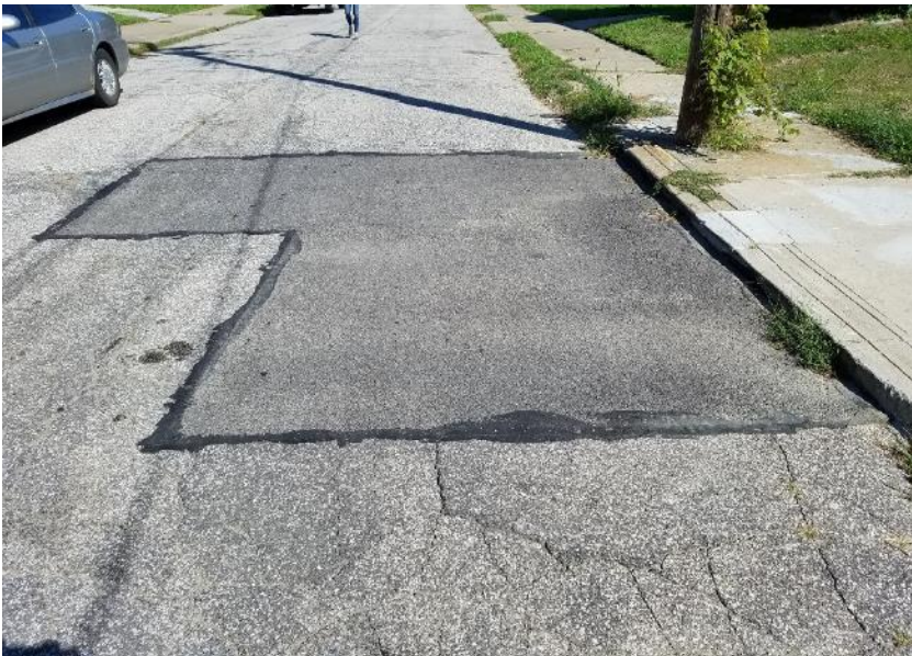
Figure 29 Repair on Sanford Ave.
