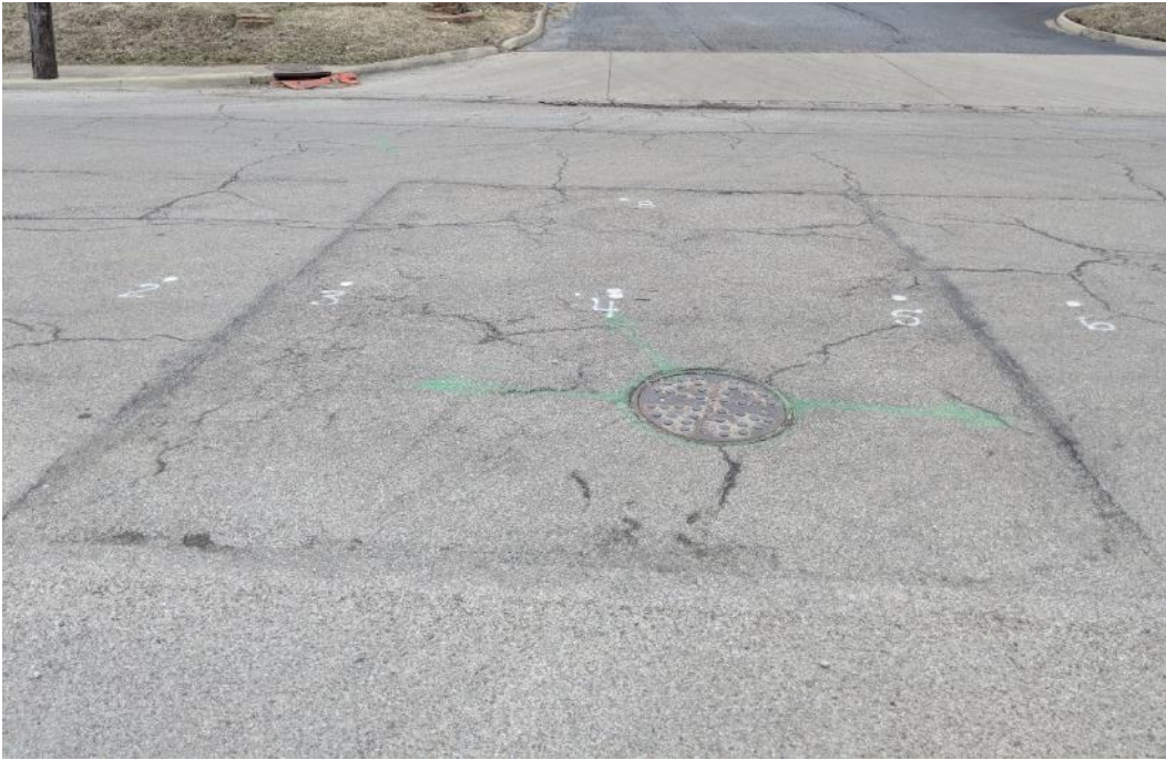
Figure 36 Repair at 1576 Old Leonard Ave.
