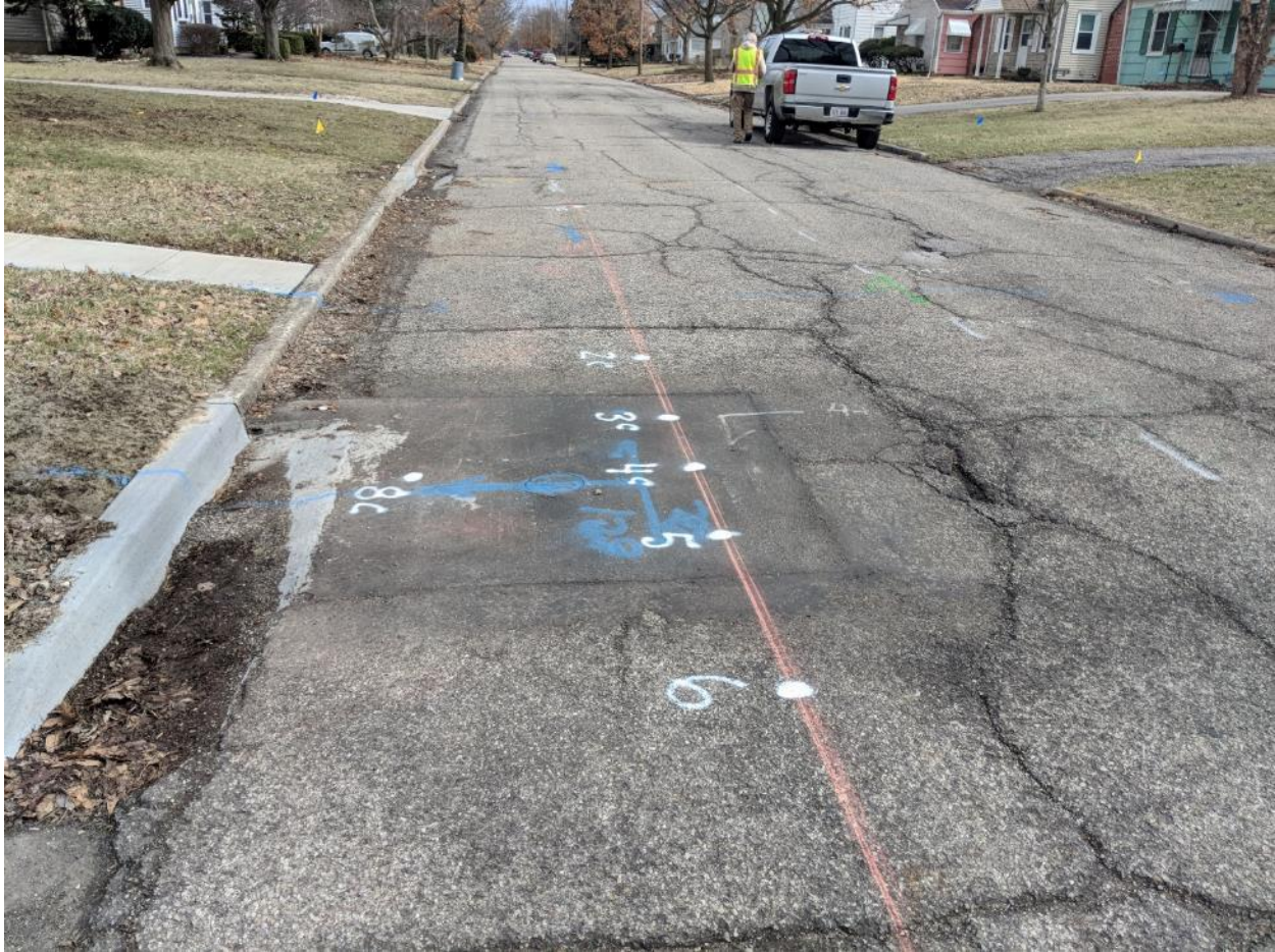
Figure 3 Example of chalk line and core layout.
