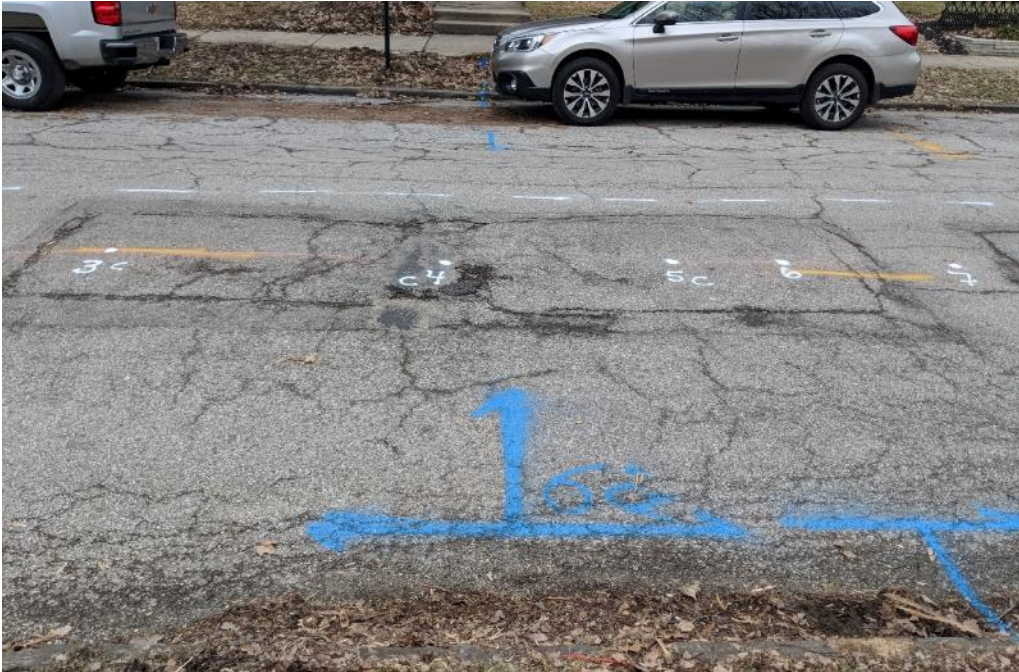
Figure 37 Repair at 61 W. 3 rd Ave.
