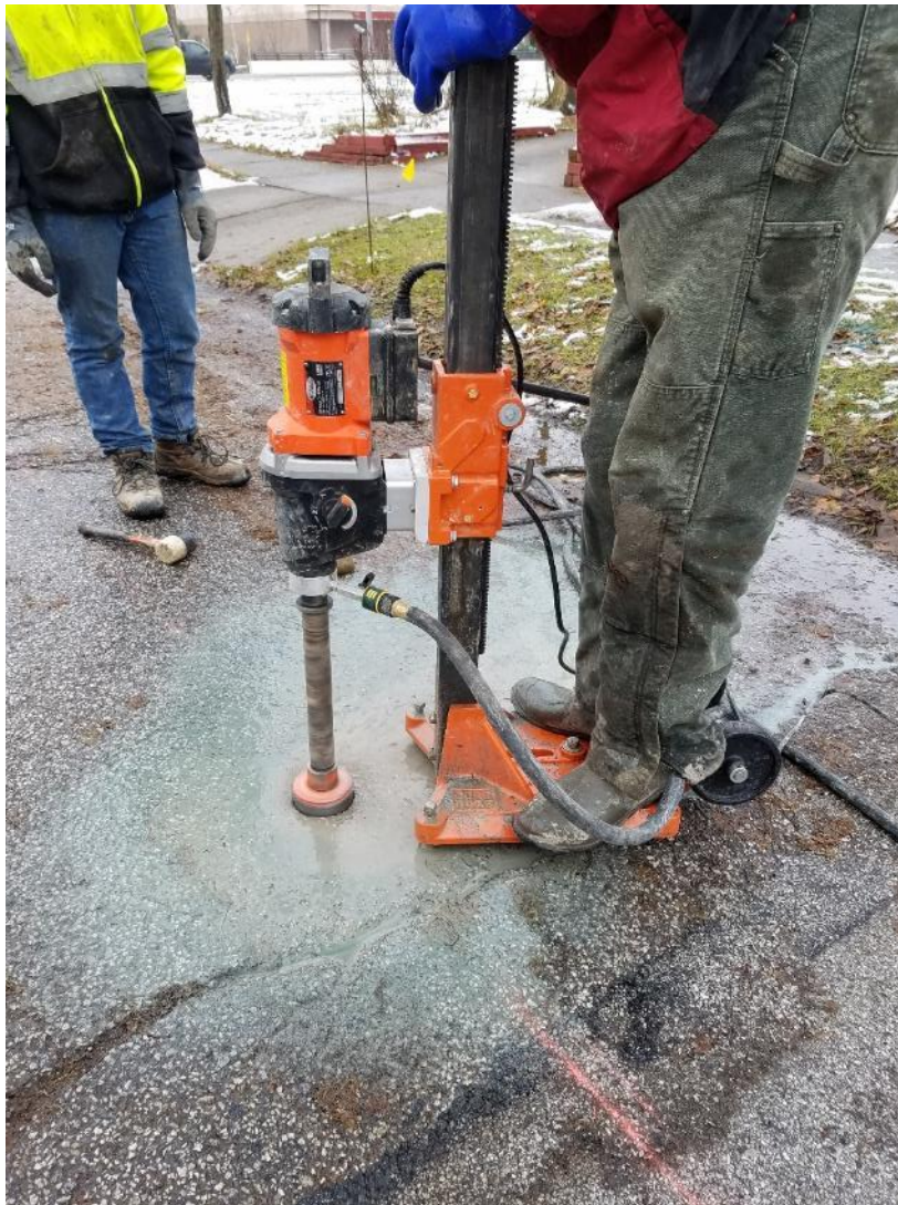
Figure 52 Coring of existing pavement.
