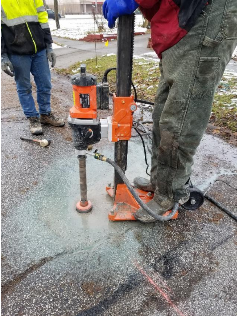
Figure 7 Coring of existing pavement.
