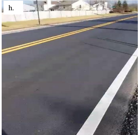
Figure B.13 Site pictures of Columbus Test Sections after Three Months of Construction: a) Control RAP Section, b) 30% RAP (64-22) Section, c) 30%RAP+SYL Section, d) 30%RAP+HYD Section, e)40% RAP+SYL Section, f) 40%RAP+HYD Section, g) 50% RAP+SYL Section, and h) 50%RAP+HYD Section
