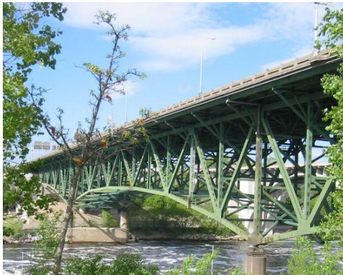
(a) Before collapse
