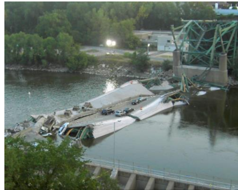
(b) After collapse
