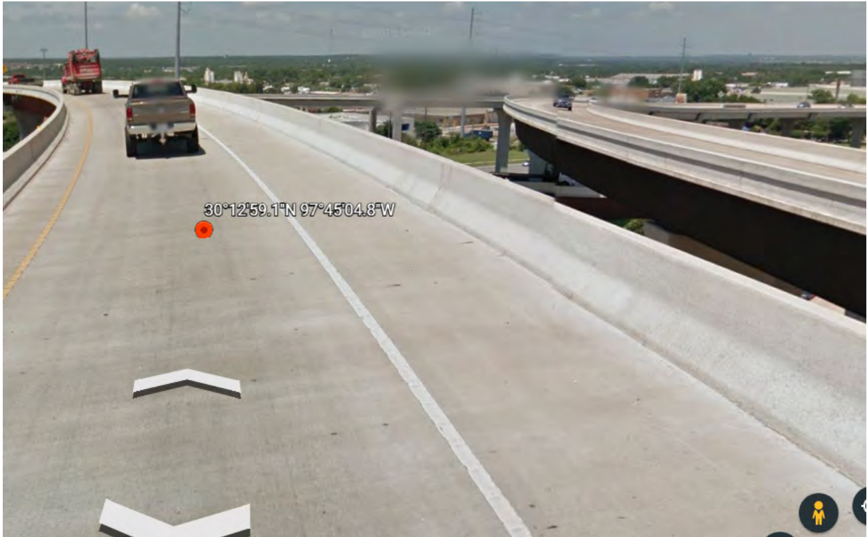
Crash Narrative 4: Driver hit curb line wall and flew over bridge; fatal.
