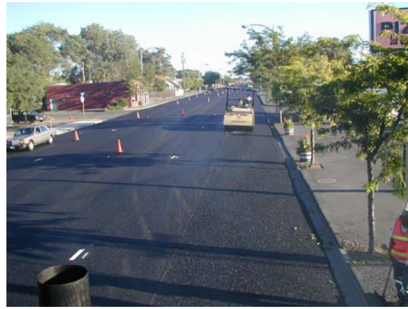
Photo 16. Compaction of the NovaChip® roadway surface.
