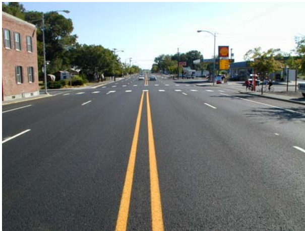
Photo 24. Soap Lake – Final NovaChip ® surface.
