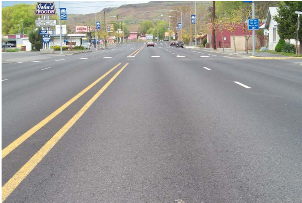
Photo 26. NovaChip® overlay through Soap Lake – May 2003.
