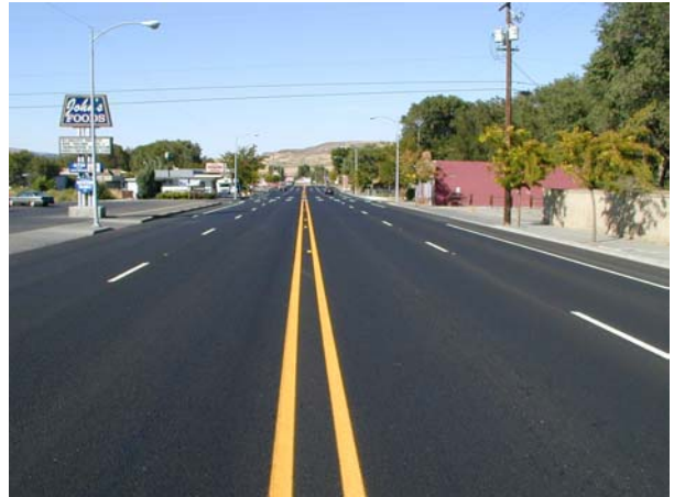
Photo 23. Soap Lake – Final NovaChip ® surface.
