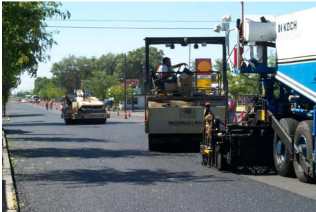
Photo 15. Rolling (seating) the NovaChip® surface.
