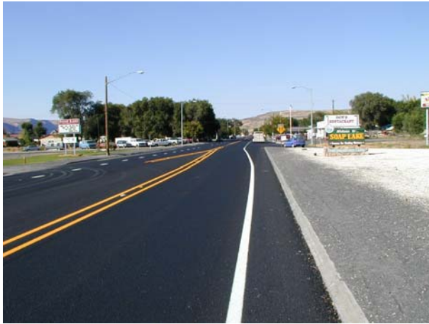
Photo 22. Soap Lake – Final NovaChip ® surface.
