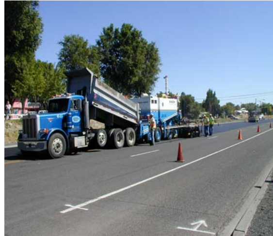
Photo 14. NovaChip® paving operation.
