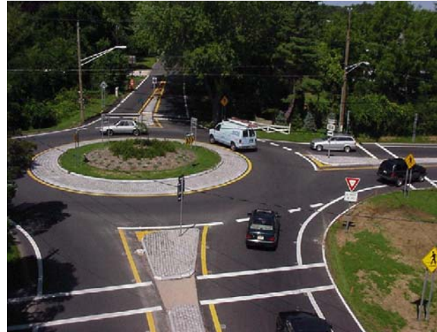
Figure 5.10 Roundabout in Suffolk County
