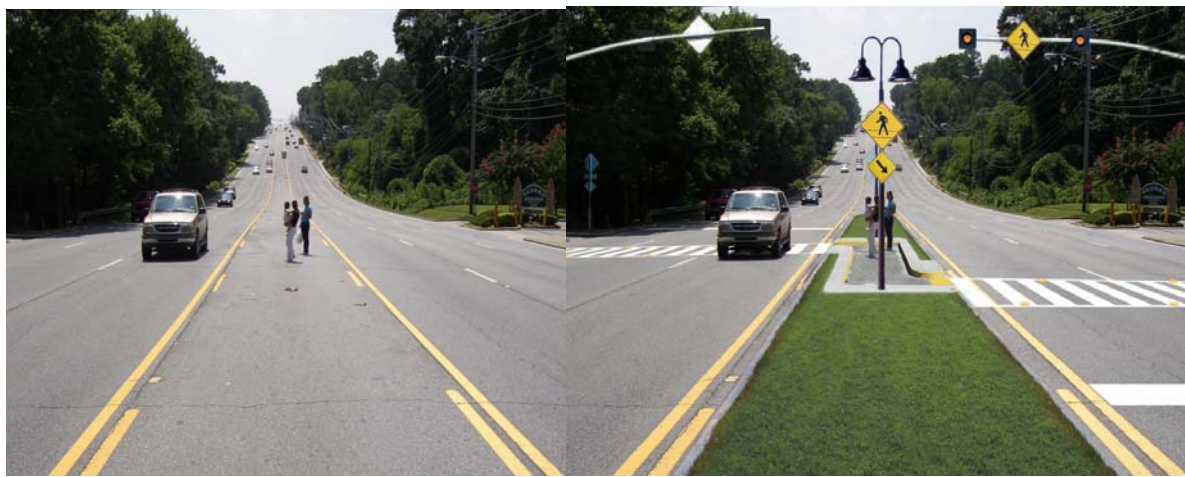
Figure 5.5 Before and After Installation of Raised Median with Slalom Path (Computer enhanced)
