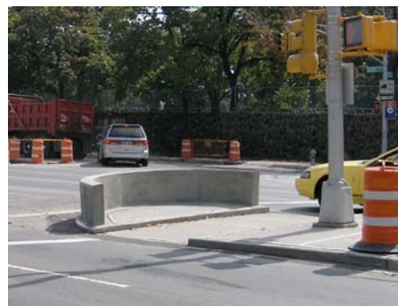
Figure 5.4 Raised Median with Non-raised Path for Wheelchairs
