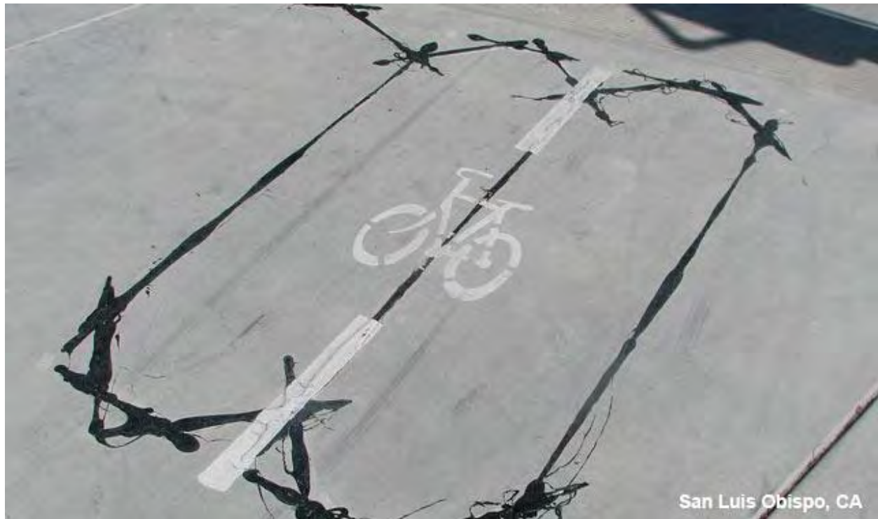
Figure 6. Example of Inductive Loop Bicycle Detector in California [5]
