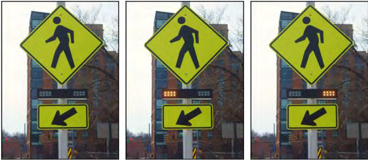
Figure 28. RRFB in Dark and Flashing Mode with W11-2 Sign and W16-7P Plaque [A.9]
