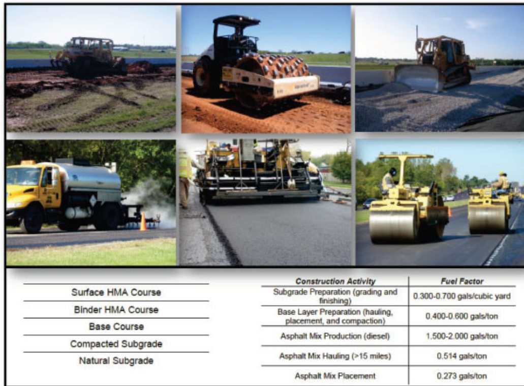
Figure 39 Paving equipment and the fuel factors [4]
