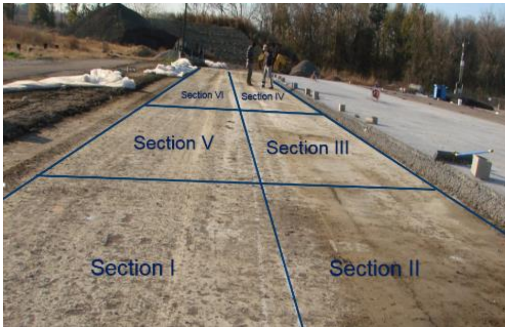
Figure 21 Overview of PRF test sections
