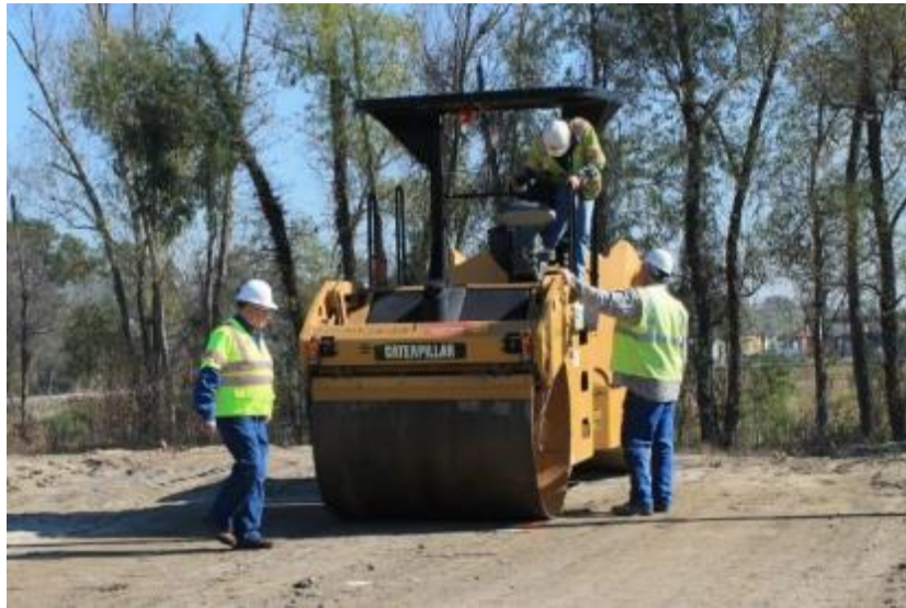
Figure 9 Roller compactor used for the micro-cracking process at PRF
