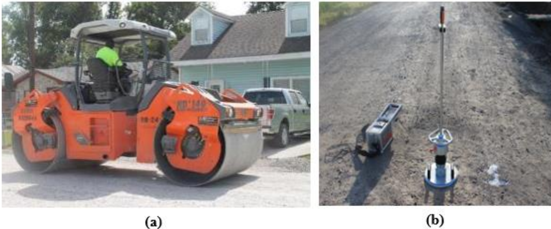
Figure 13 (a) Roller for micro-cracking (b) LFWD used on LA1003
