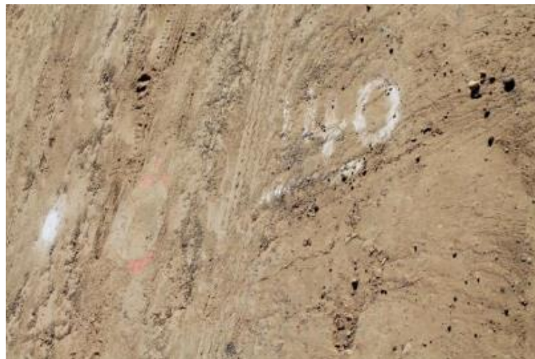
Figure 16 Micro-cracking with vibratory roller (HD 140)
