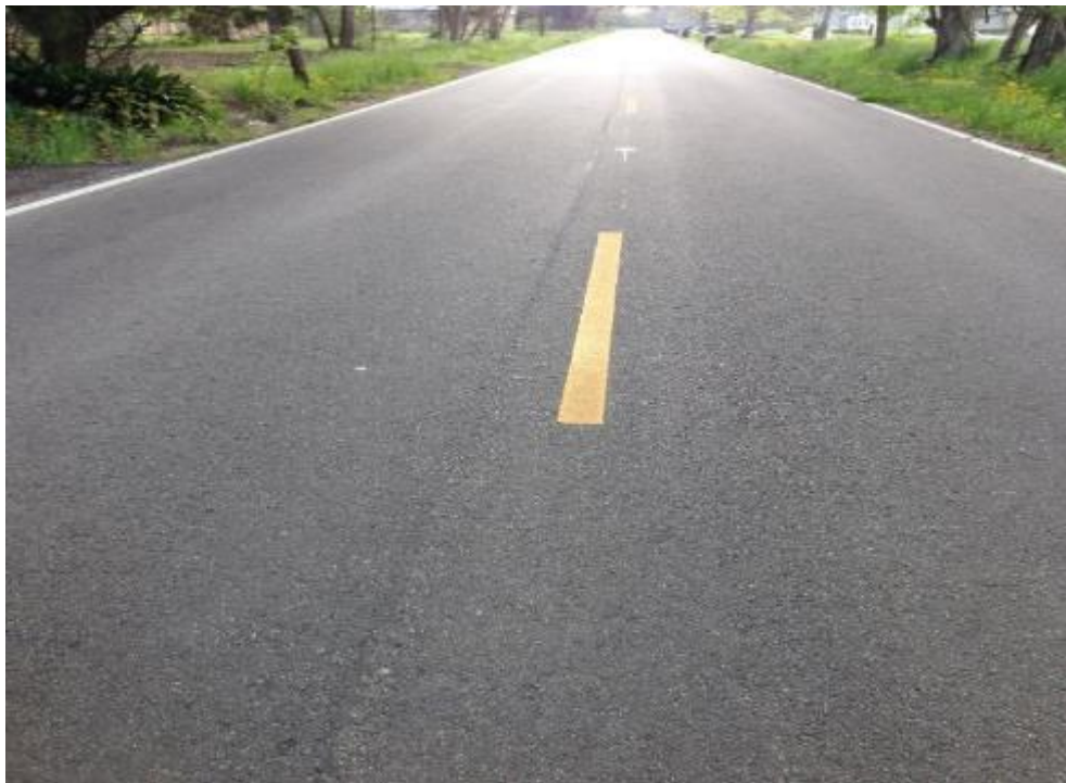
Figure 31 Eastside view of Section I on LA1003
