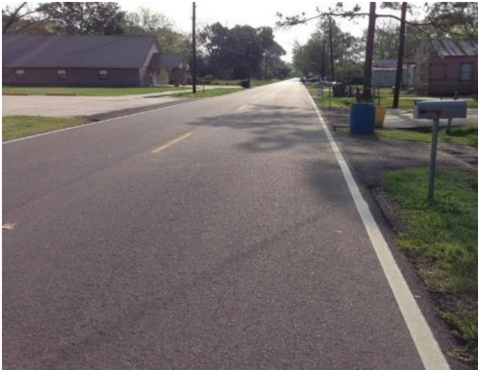
Figure 33 Westbound lane of Section II (second part) on LA1003
