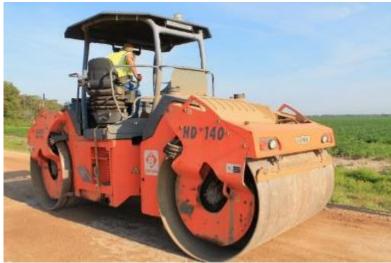
Figure 16 Micro-cracking with vibratory roller (HD 140)
