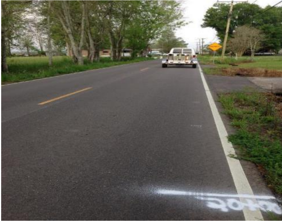
Figure 32 Westbound lane of Section II (first part) on LA1003
