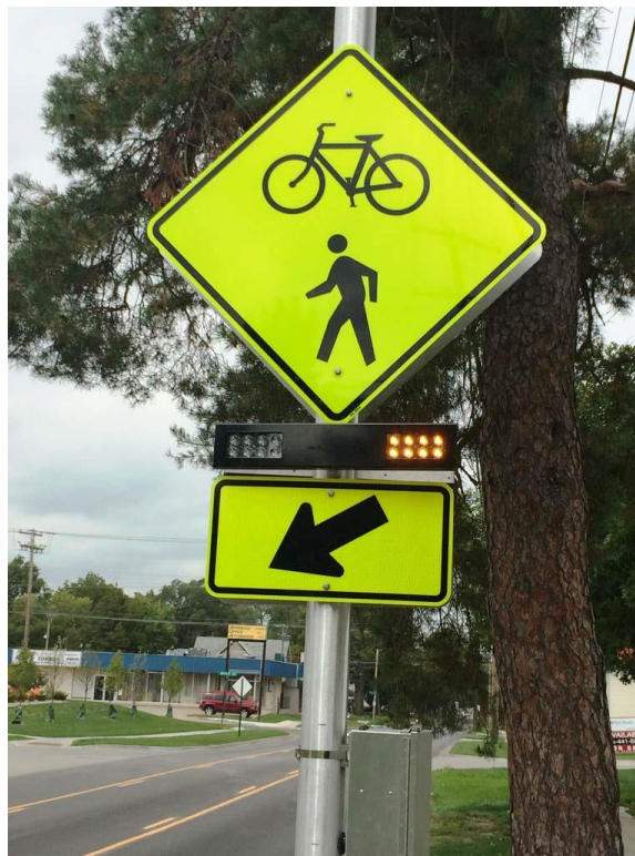
Figure B8. Rectangular rapid flashing beacon
