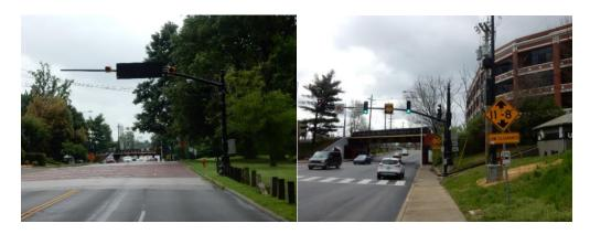
• **KY 1136 in Hardin County between KY 1868 and US 31W:** Truck prohibition signs were placed along a section of this roadway. The prohibition is a result of low ground clearance railroad crossing in this section of KY 1136.
