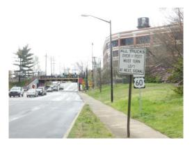
• Install warning signs in advance of low ground clearance railroad crossings.
