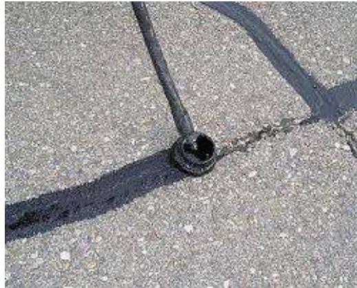
Figure 1 Typical crack sealing application
