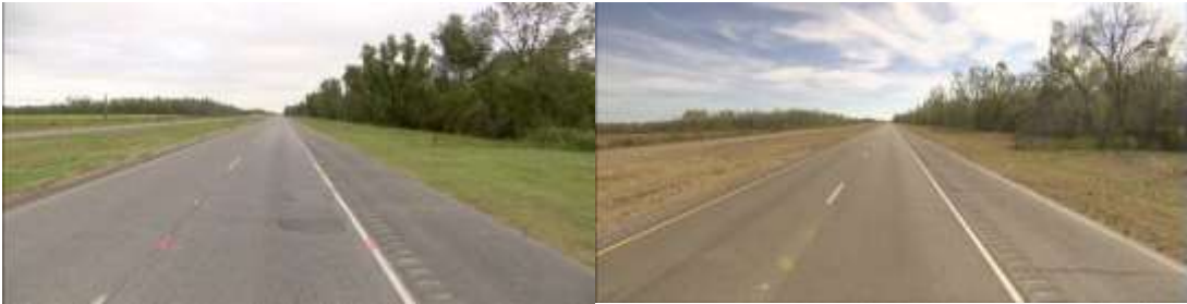
Figure 35 Pavement section before (left) and after (right) microsurfacing
