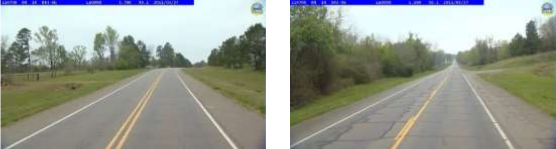
Figure 33 Pavement section before (left) and after (right) crack sealing
