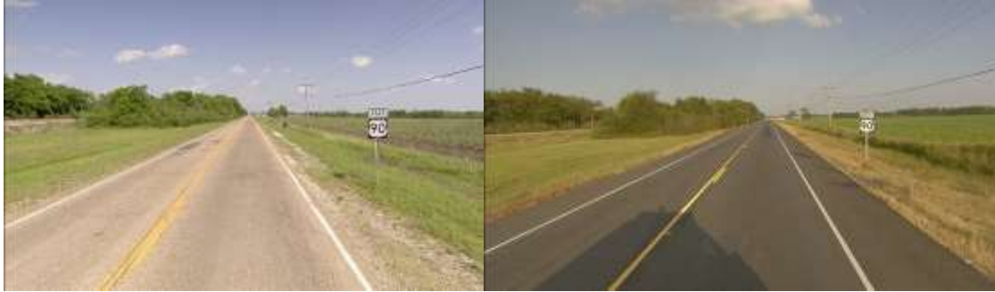
Figure 36 Pavement section before (left) and after (right) AC overlay
