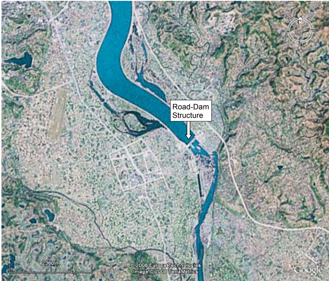
Figure 9: Satellite optical image of the city of Mianyang in Sichuan province, China, which was impacted by the 2008 earthquake.
