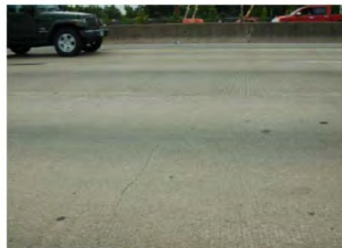
Transverse cracks
