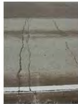
Picture 4 Area of potential punchout (RM 51 + 214 ft)
