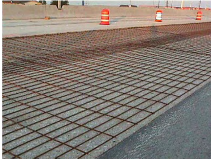
Figure 3.2: Steel placed directly on top of substrate
