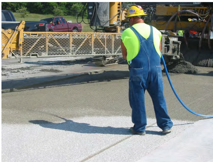
Figure 3.3: Spraying grout immediately ahead of paver
