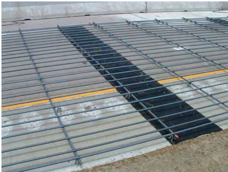
Figure 8.4: Prepared surface prior to the yellow stripe removal
