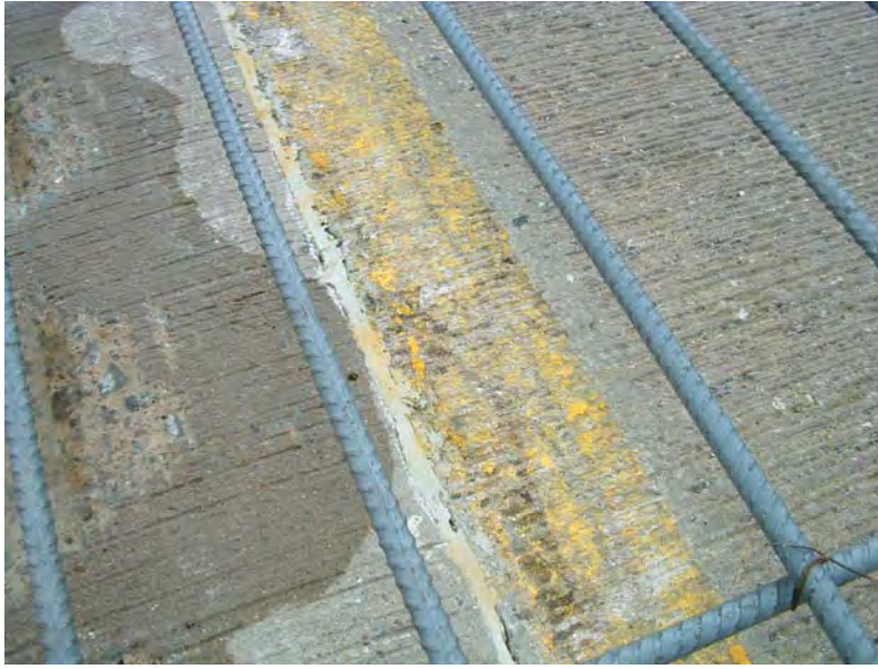
Figure 8.5: After the removal of the yellow stripe
