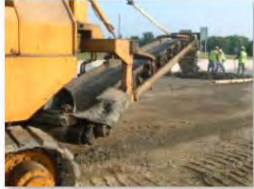
Start of Construction
