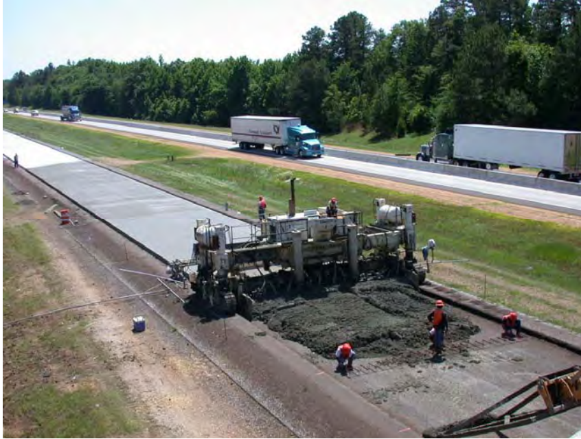
Figure 5.5: Prompt curing following the paver
