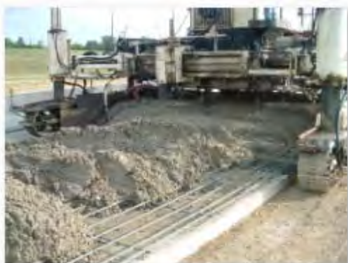
Ahead of the Paving Machine
