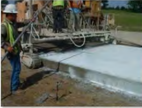
Spraying Curing Compound
