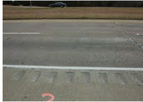
JCP slab in good condition
