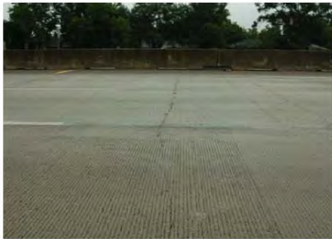
Transverse cracks
