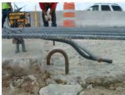
Close-Up of Reinforcement at Transition
