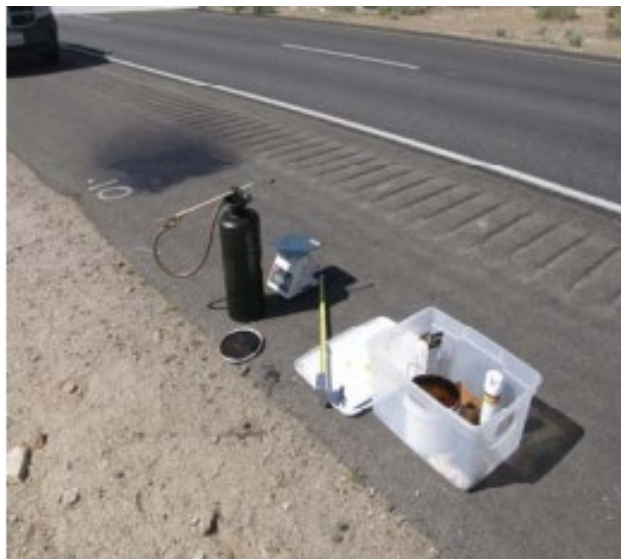
Figure 3. Visual method of determining pavement emulsion absorption capacity (Caltrans).
