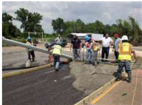
(b) Pouring of concrete
