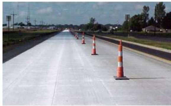
(b) New constructed UTW section on US65 (19)
