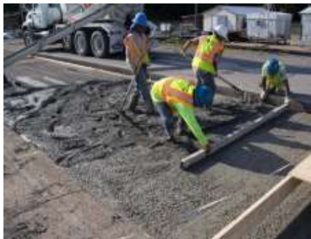
(c) Placement of concrete
