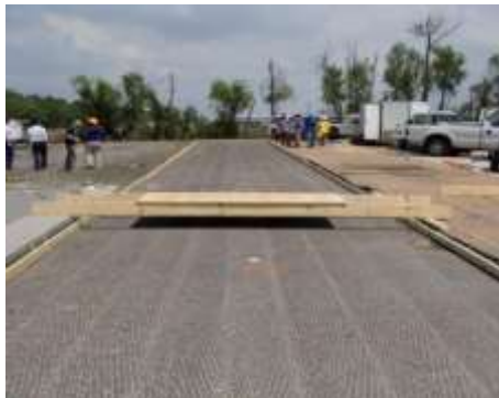
(a) Milled asphalt
