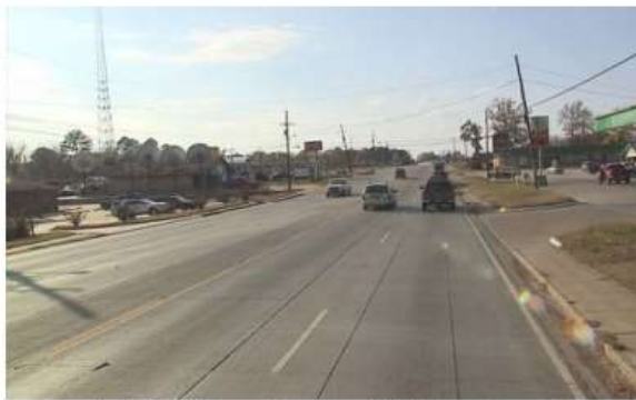
(a) UTW section on US167 after 13.5 years of service
