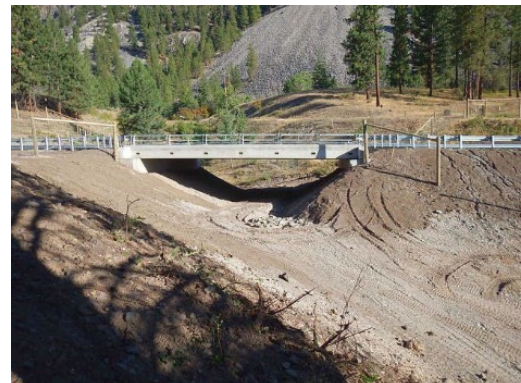
Photo 1. Underpass built for Rocky Mountain bighorn sheep, Hwy 200 East of Thompson Falls, MT.
