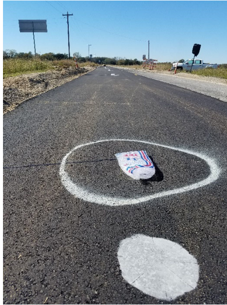
Figure 8 Typical asphalt test site
