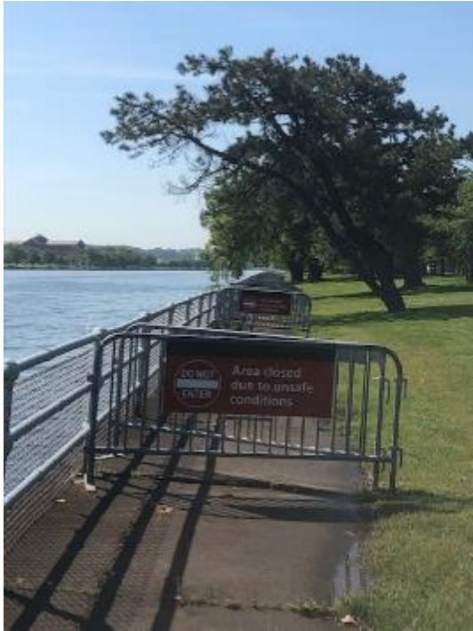
FIGURE 7: CLOSED SEAWALL PEDESTRIAN PATH AT HAINS POINT (VOIGT, 2021)
